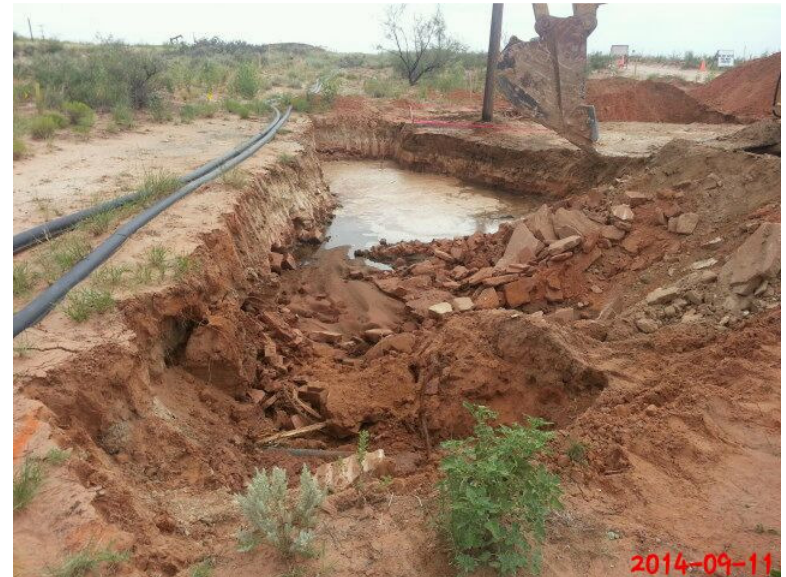
Initial release in south excavation caused by struck fiberglass line, facing south 9/11/14
