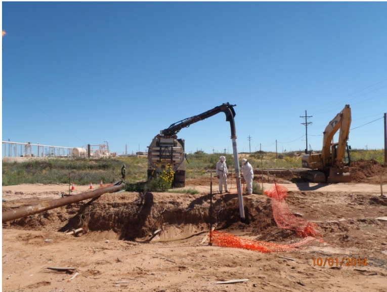
Hydro-excavating wet material from north excavation, facing east 10/1/14
