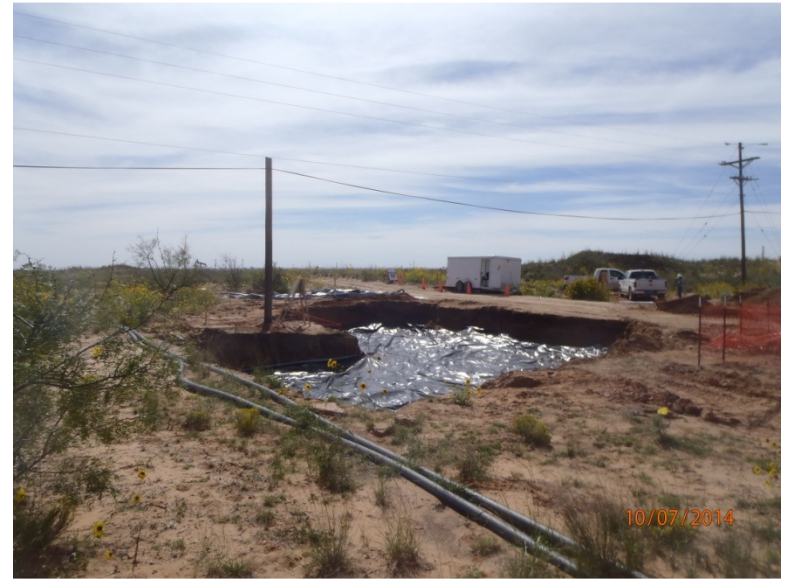
Liner installation in south excavation completed, facing southwest 10/7/14
