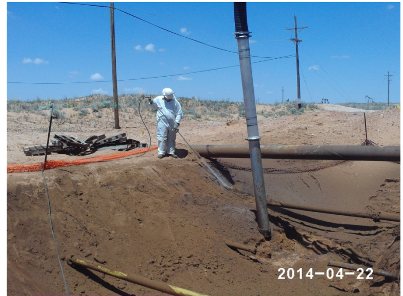
Hydro-excavating north release area, facing northwest 4/22/14
