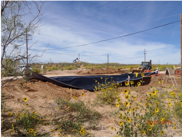
Installing liner in south excavation, facing northwest 10/7/14
