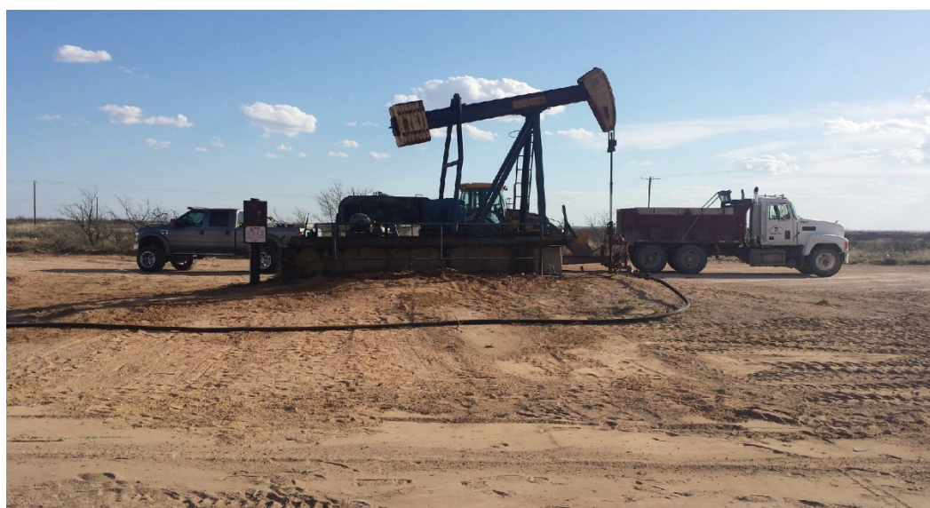
Completed site with contaminated dirt hauled out, blended caliche leveled back in
