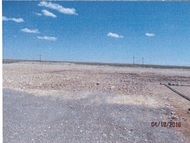
This photo was taken 4/16/2015 after the location had been scraped with a box blade and rippers and sprayed with a microblaze solution. This photo was taken near the Date BTB State Com #4H wellhead and is looking to the east.
