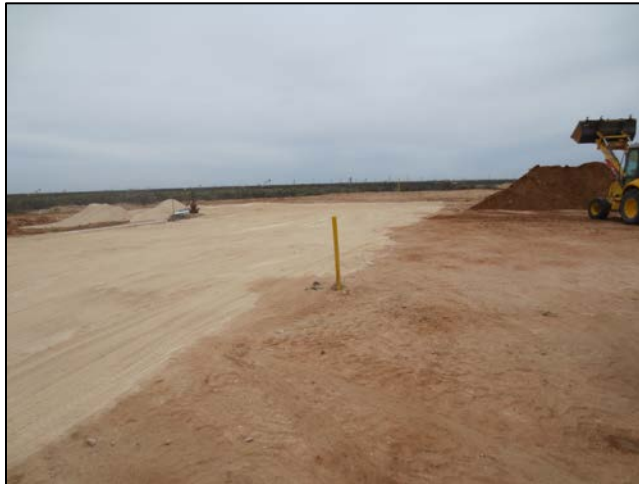
Backfill of wellhead area
