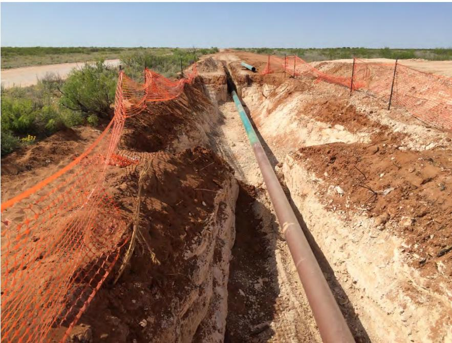
Pipeline excavation exposing a 10-15 foot thick caliche bed near the proposed containment.
