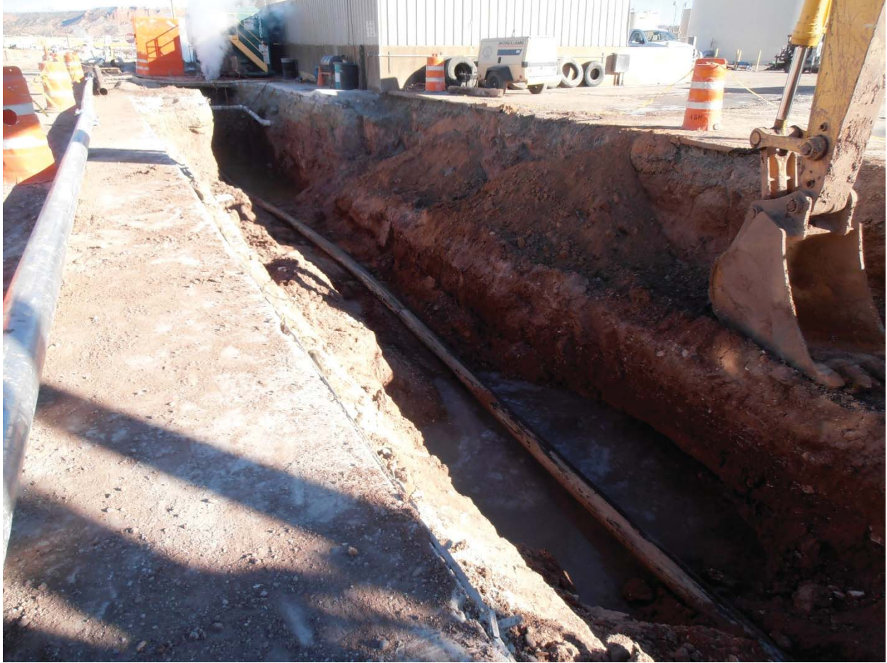
View of excavation looking to north with Bundle Cleaning Pad in background.
