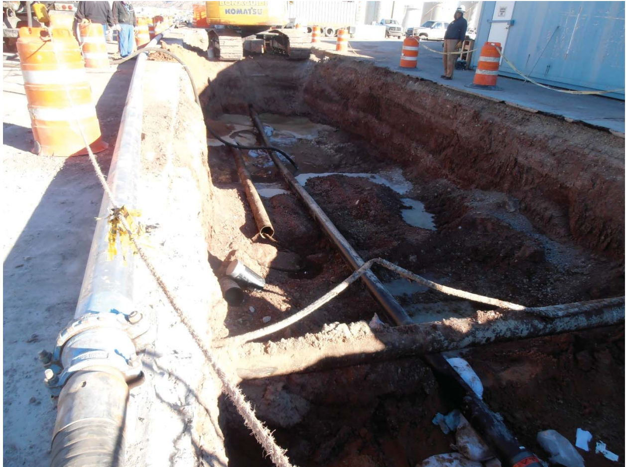
View from south end of excavation looking to the north.
