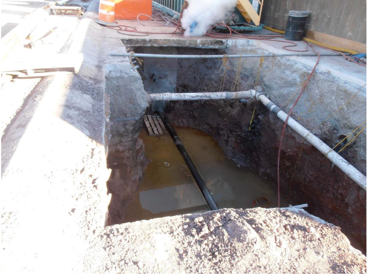
View of north end of excavation with new sewer line terminating into concrete sewer junction box on west side of Bundle Cleaning Pad.
