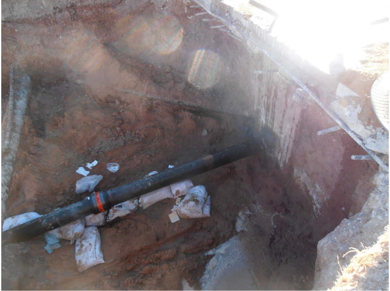
Photo of south end of excavation looking to the east. South wall is concrete sewer junction box.
