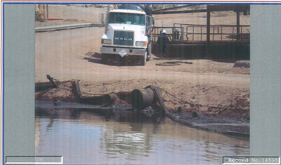
AL1 pipes - (left - drain for bermed area) (right - from old API separator to AL1)
