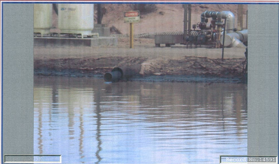
AL1 pipe - API separator water section overflow.
