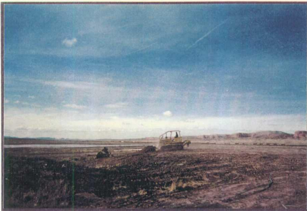
Soil Layer Placement
