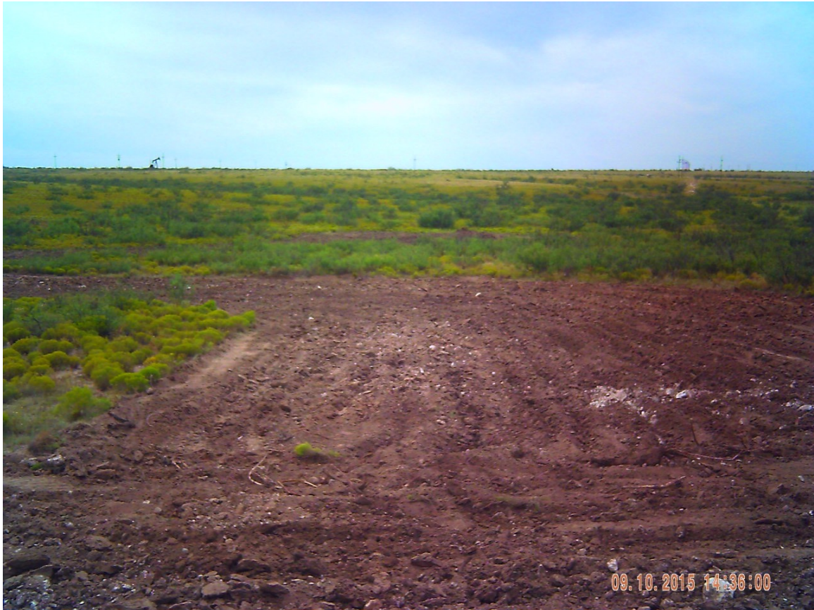
Standing on West end of well pad-looking SW- Area plowed, disked and fertilized.
