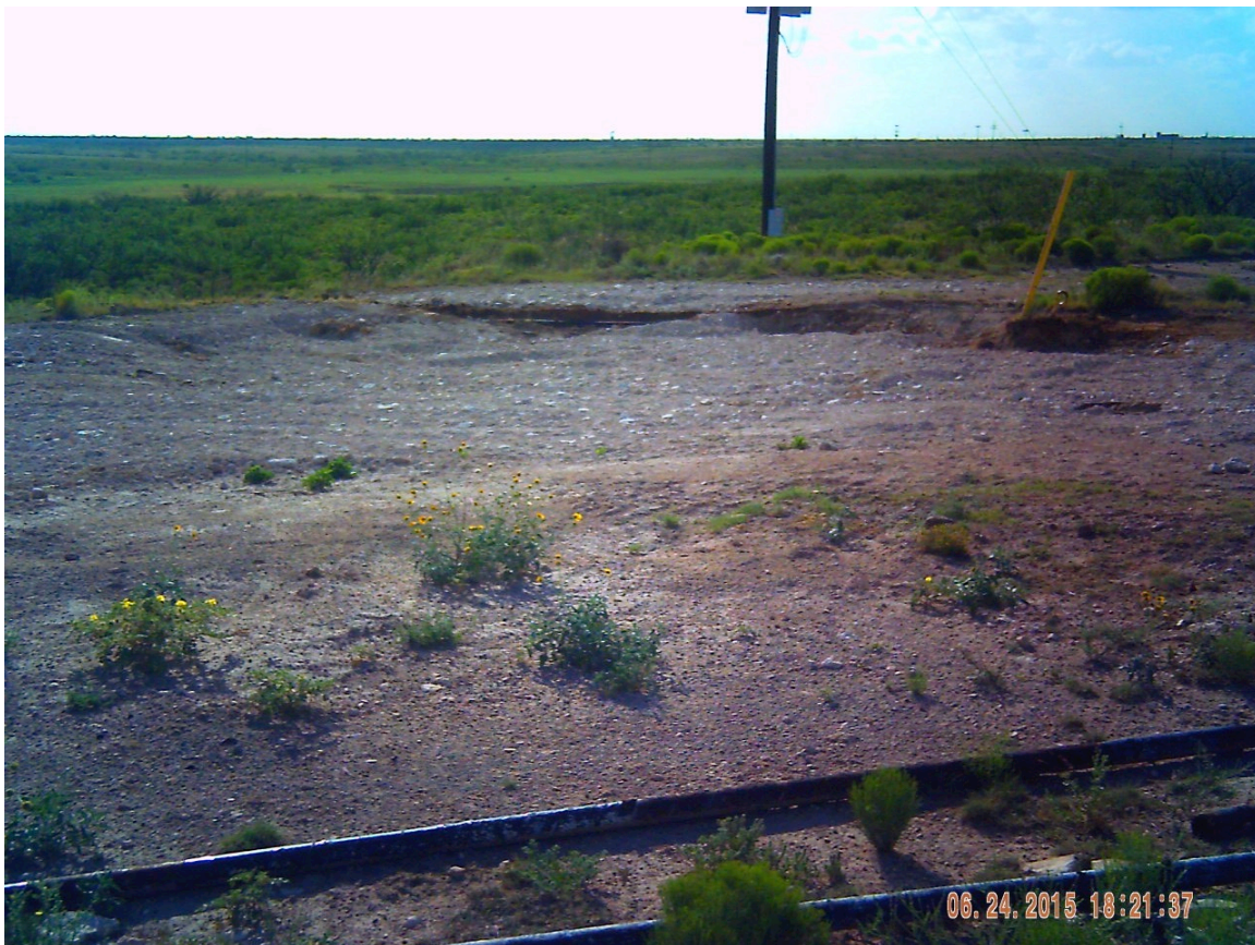
Pool #5 Pad Area Looking West, background shows Playa Lake and Cattle Pond.- This area was excavated to remove oily stained soil and sampled.
