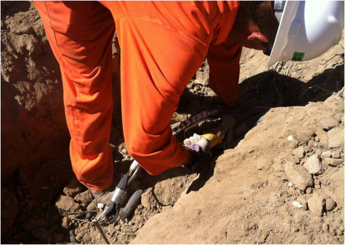
Removal of electrical conduits.
