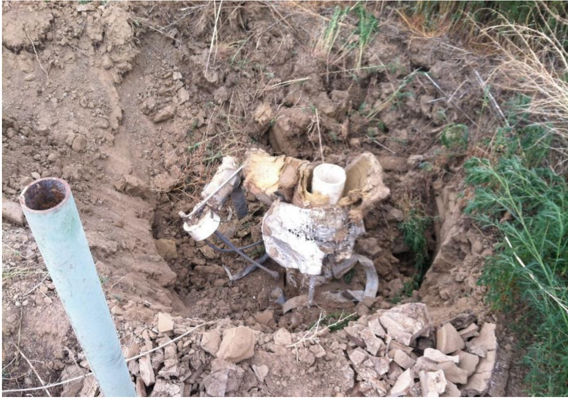
Removal of equipment at air sparge well.
