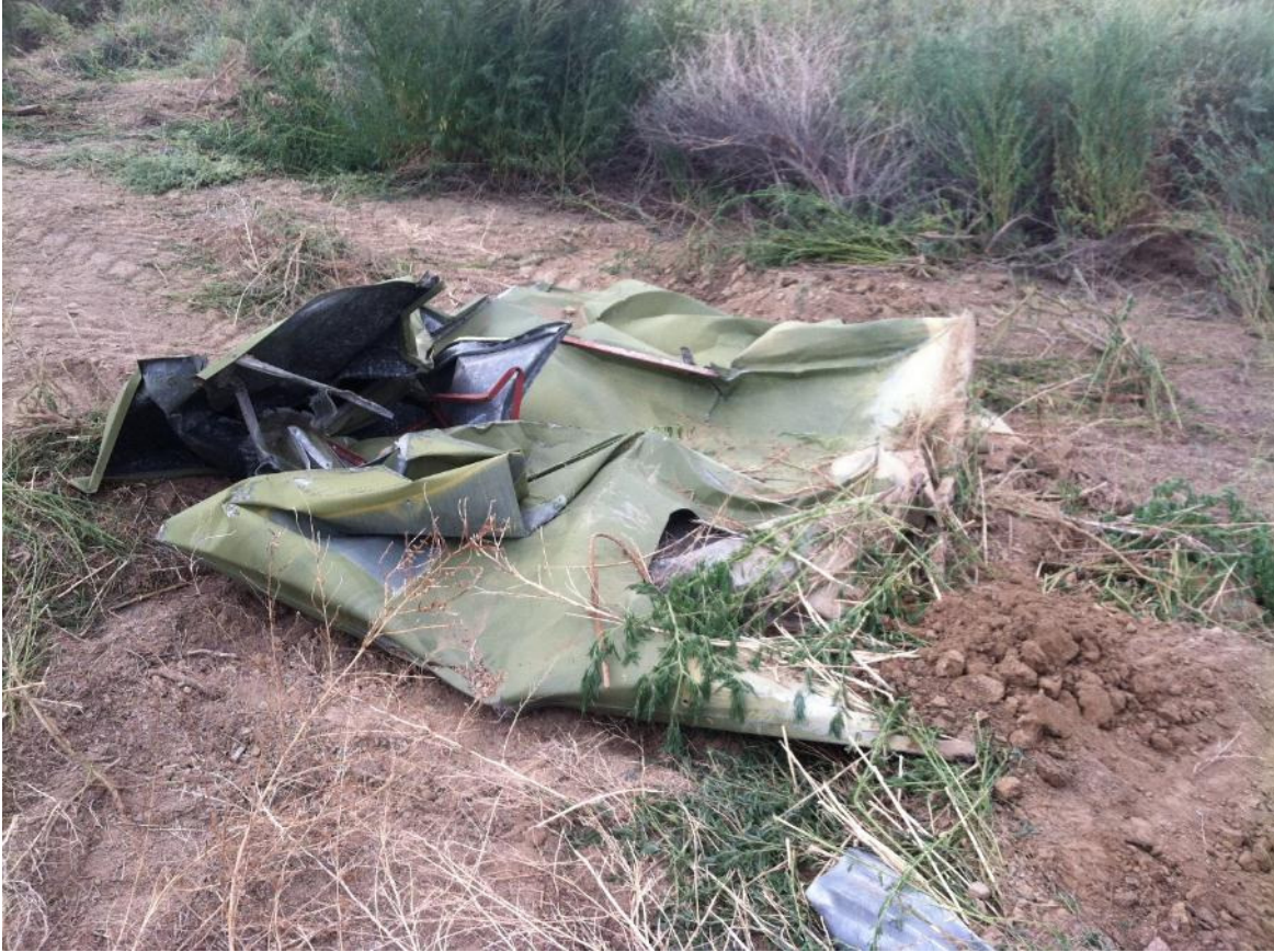
Demolition of secondary shed for air sparge system.
