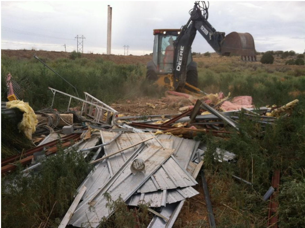
Demolition air sparge system shed.
