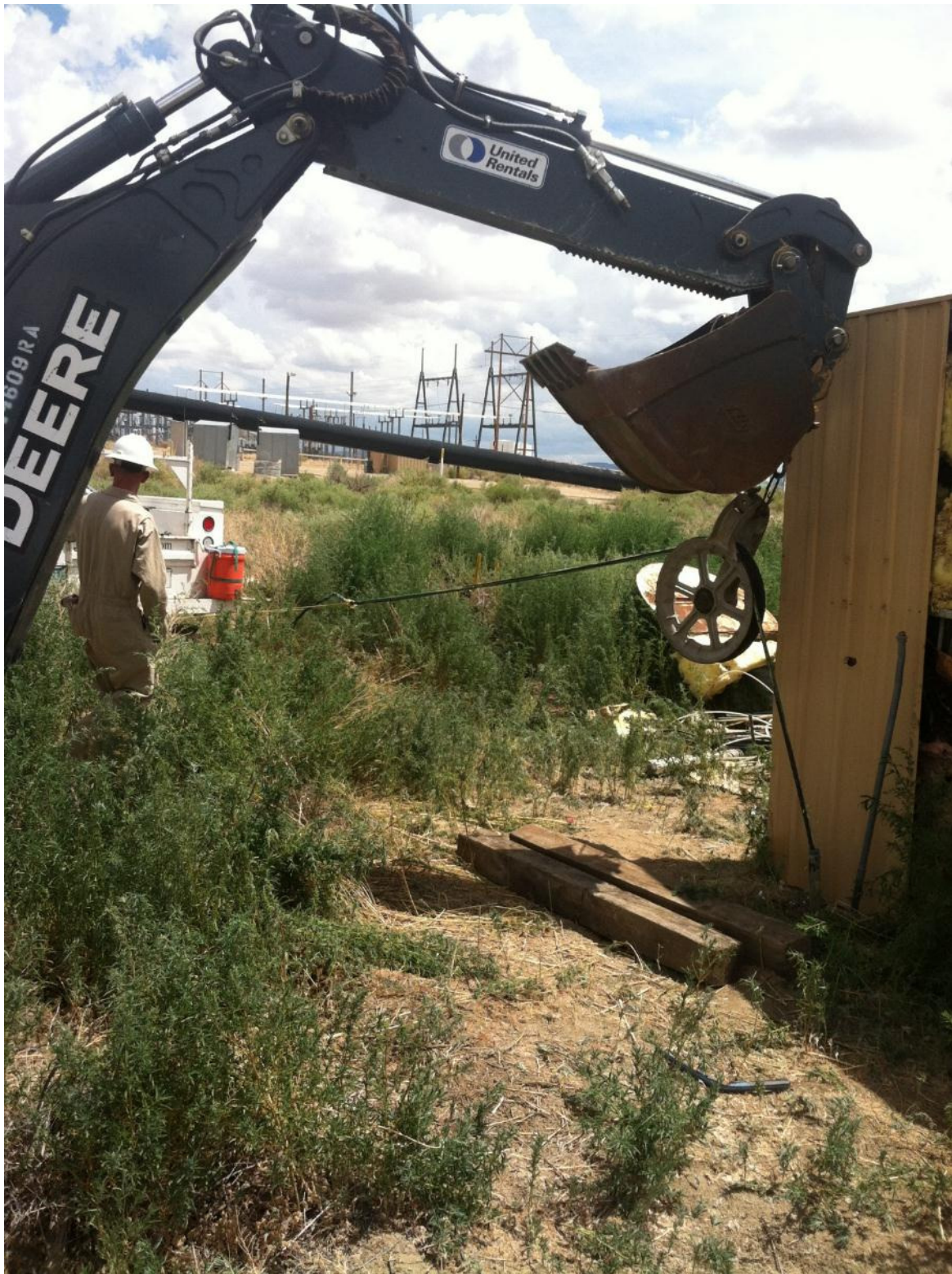
Removal of electrical conduit/wiring supplying power to air sparge system shed.
