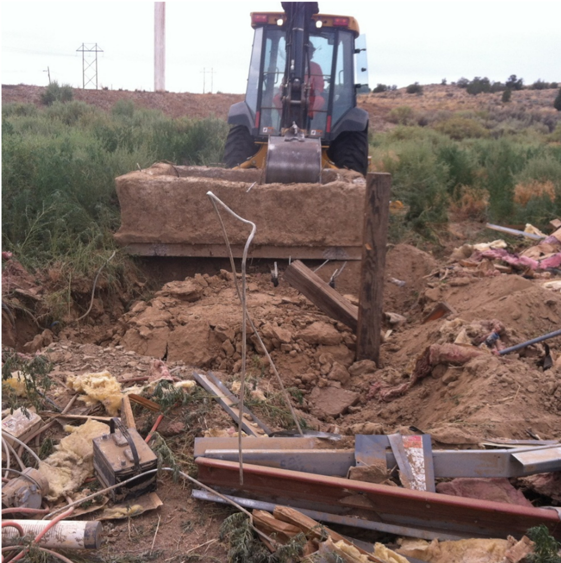
Demolition of air sparge storage shed.
