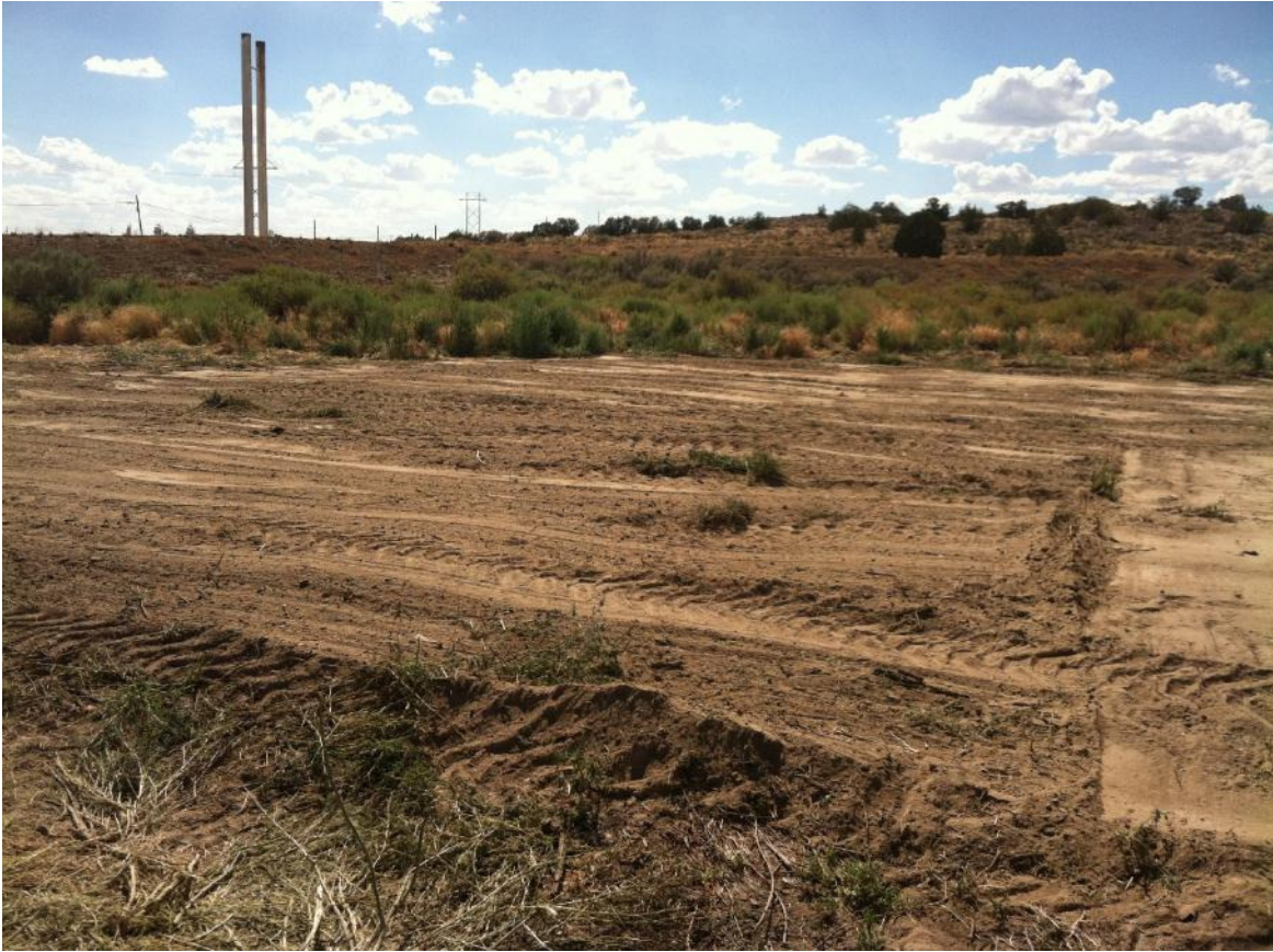
Completion of grading at location of former sir sparge system storage shed.
