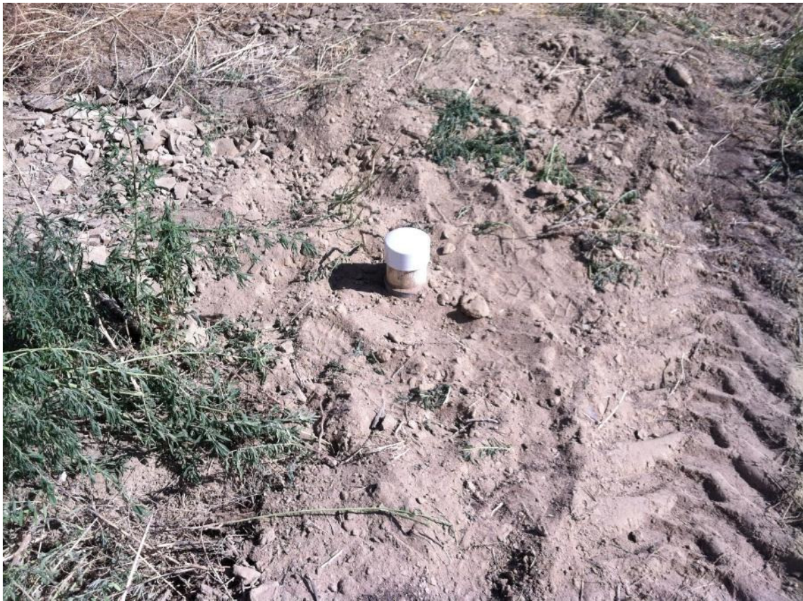
Equipment demolition complete at air sparge well.
