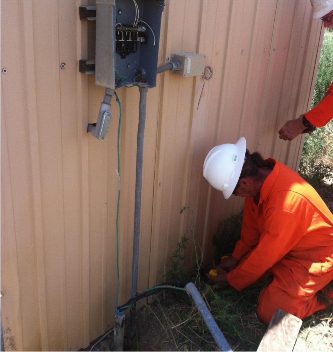
Demolition of air sparge system storage shed.
