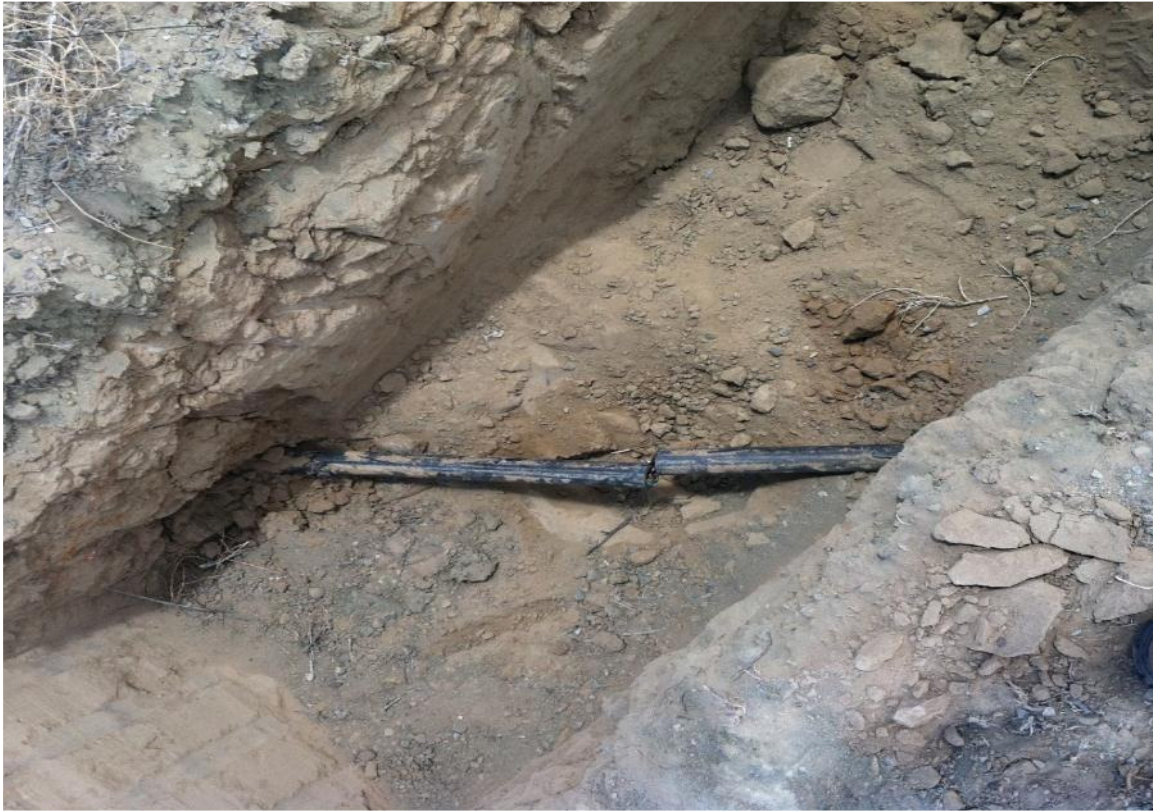
Termination of power supply to air sparge system shed.
