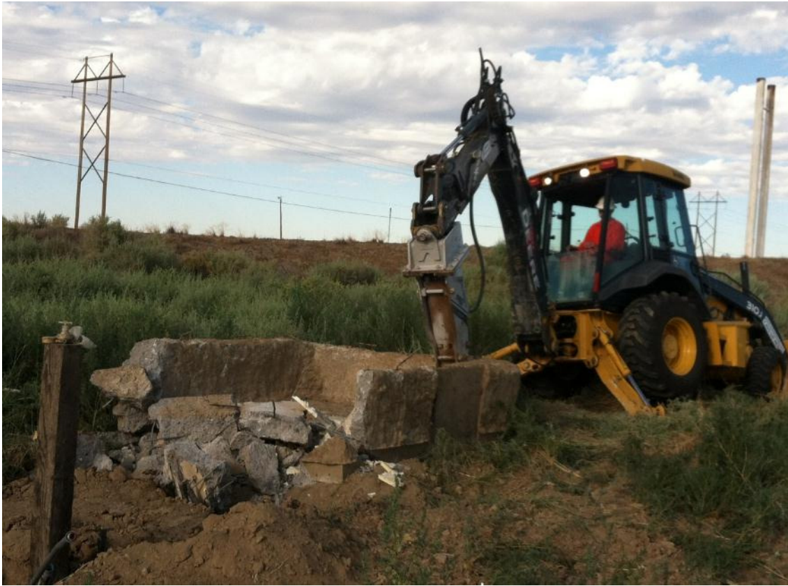
Demolition of air sparge storage shed foundation.
