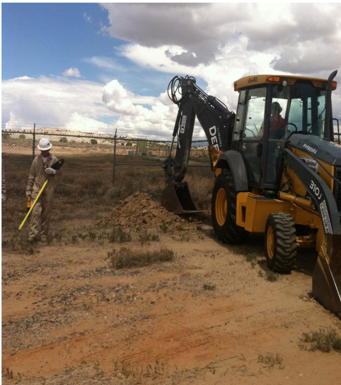
Termination of power supply to air sparge system shed.
