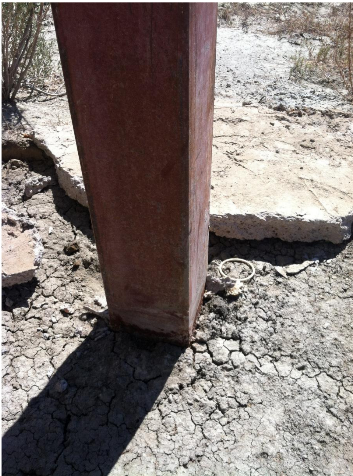
Concrete pad removal at MW-32.
