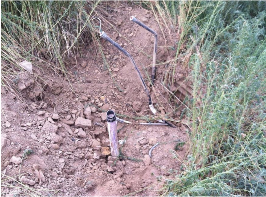
Removal of electrical conduits.
