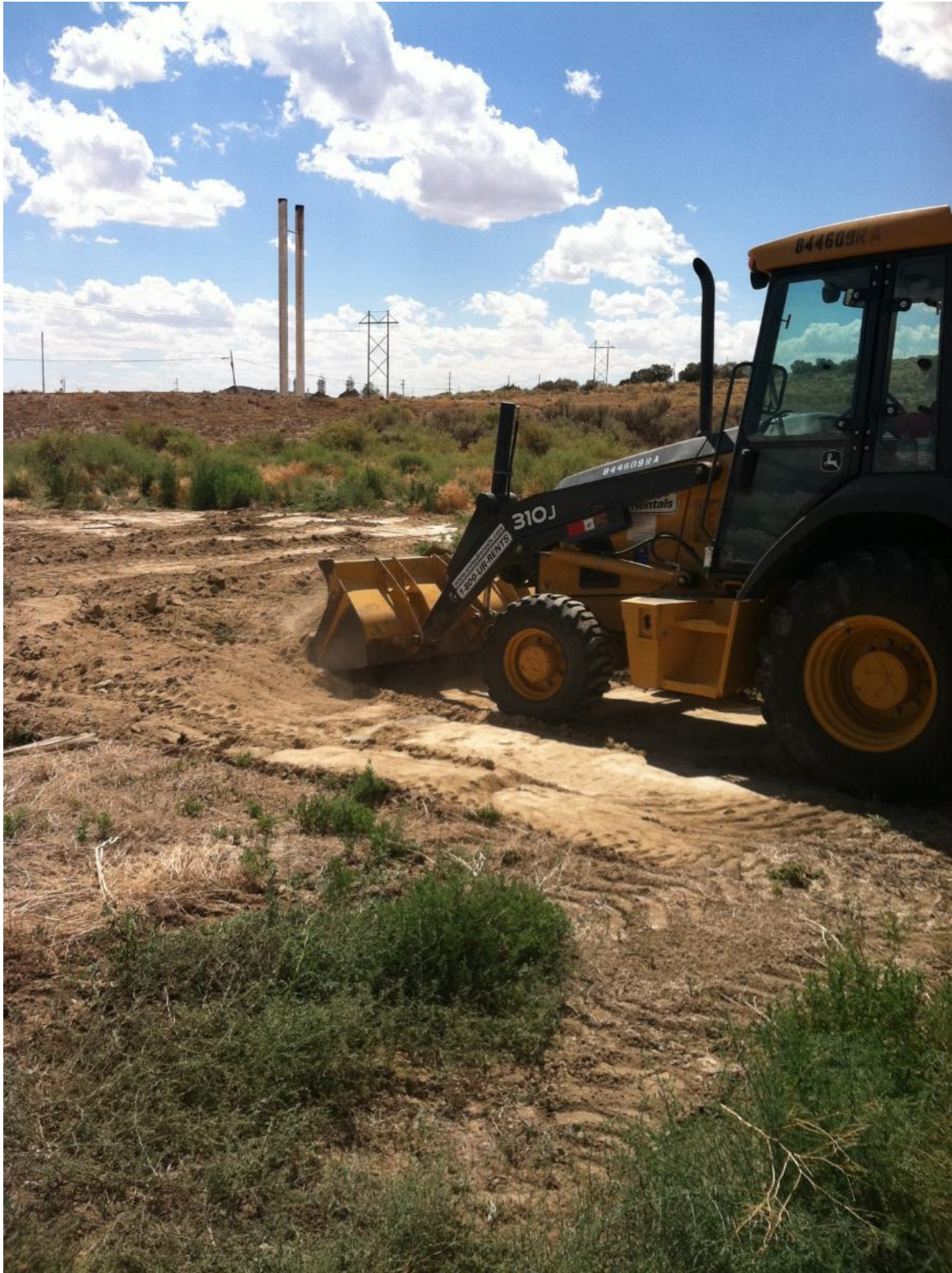
Grading location of former air sparge storage shed.
