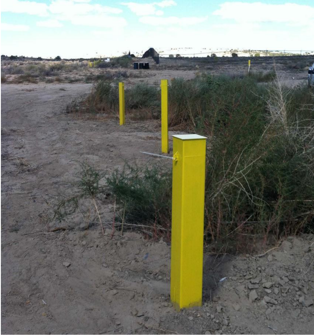
Installation of steel protective stick-ups for MW-19, MW-27, and SW-1.
