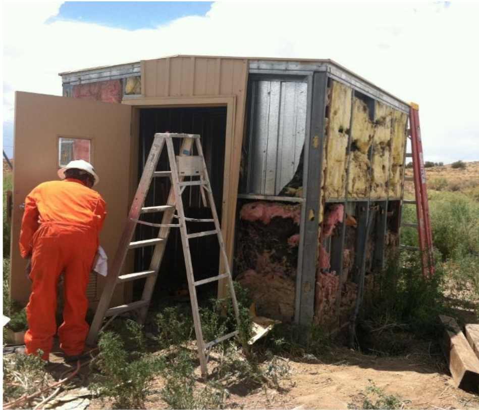
Demolition of air sparge storage shed.
