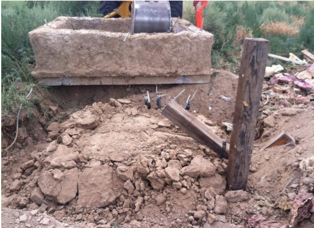
Demolition of air sparge storage shed.
