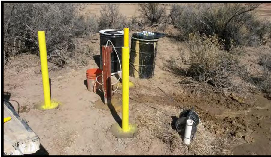
Photo 6: Purging the completed monitor well (MW-1) with a Grunfos submersible electric pump, after wells where surged with a PVC slug. Field parameters where measured with a calibrated HACH meter (on barrel) to monitor stabilization of pH, Temperature and Conductivity.
