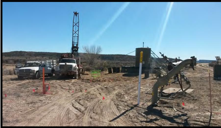
Photo 3: Enviro-Drill Inc. from Albuquerque installed the boreholes and monitor wells on site using a CME-75 drill rig with Hollow Stem Auger tooling and a split spoon sampler.
