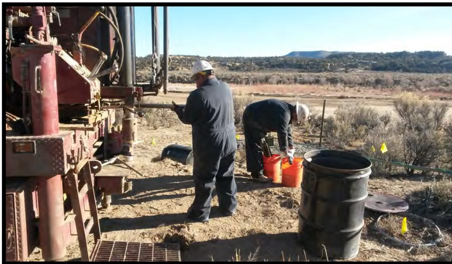
Photo 4: Split spoon sampler was decontaminated between each sample. All cuttings were drummed on site and disposed of by Envirotech.
