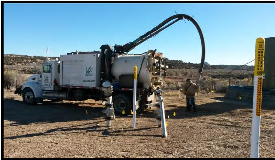
Photo 2: NRE Field Services hydro excavated the pipeline and advanced the borehole locations beyond the depth of any possible buried infrastructure. .
