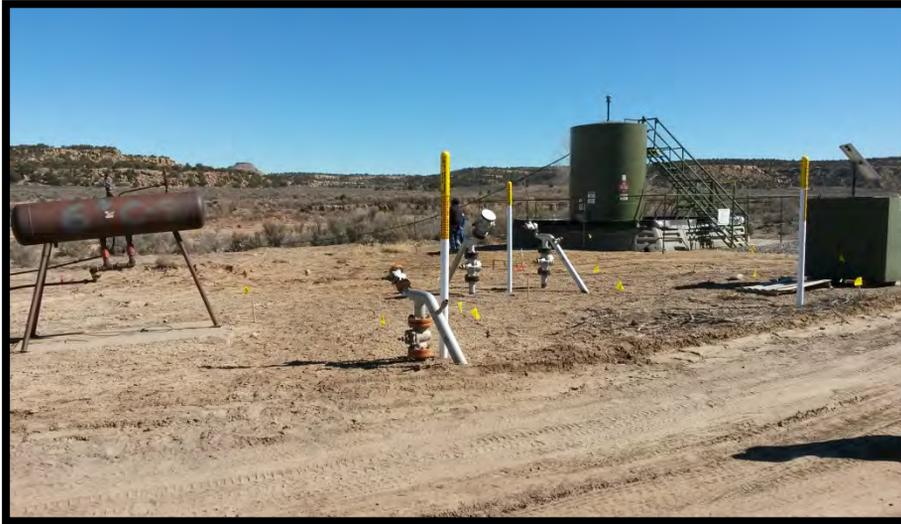
Photo 1: Lateral C-64 pipeline release site. The density of utilities and pipeline infrastructure on site constrained the well construction to proceed from farthest to closest to the road.
