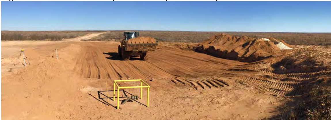
Figure 5 – The last load of suspected salt-impacted soil is placed on the level remediation cell
