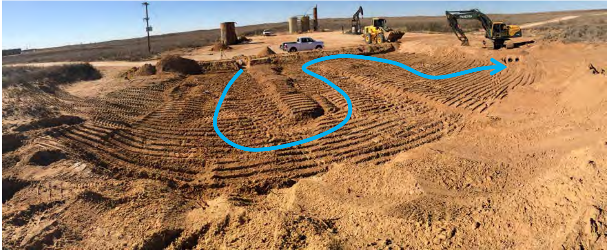
Figure 6 – As the salt soil was exhausted, a thin layer of clean soil was placed over the salt-impacted soil and stained soil to form a top bed of sand that would be suitable for seeding and growth of native plants. Berms will direct water as shown by the blue arrow from the inlet to the outlet.
