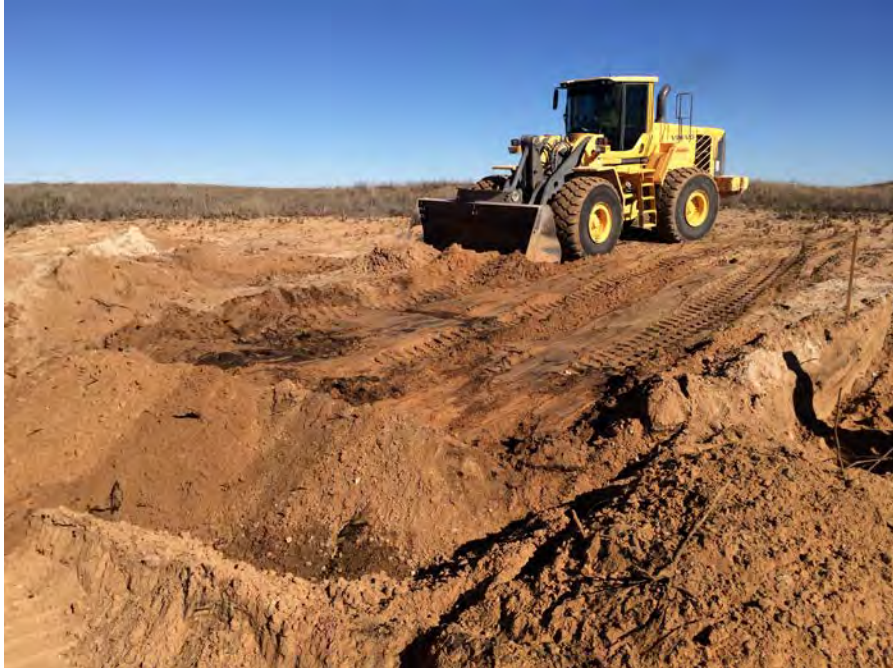
Figure 2 – Segregation of stained soil from clean soil using the best tools available.
