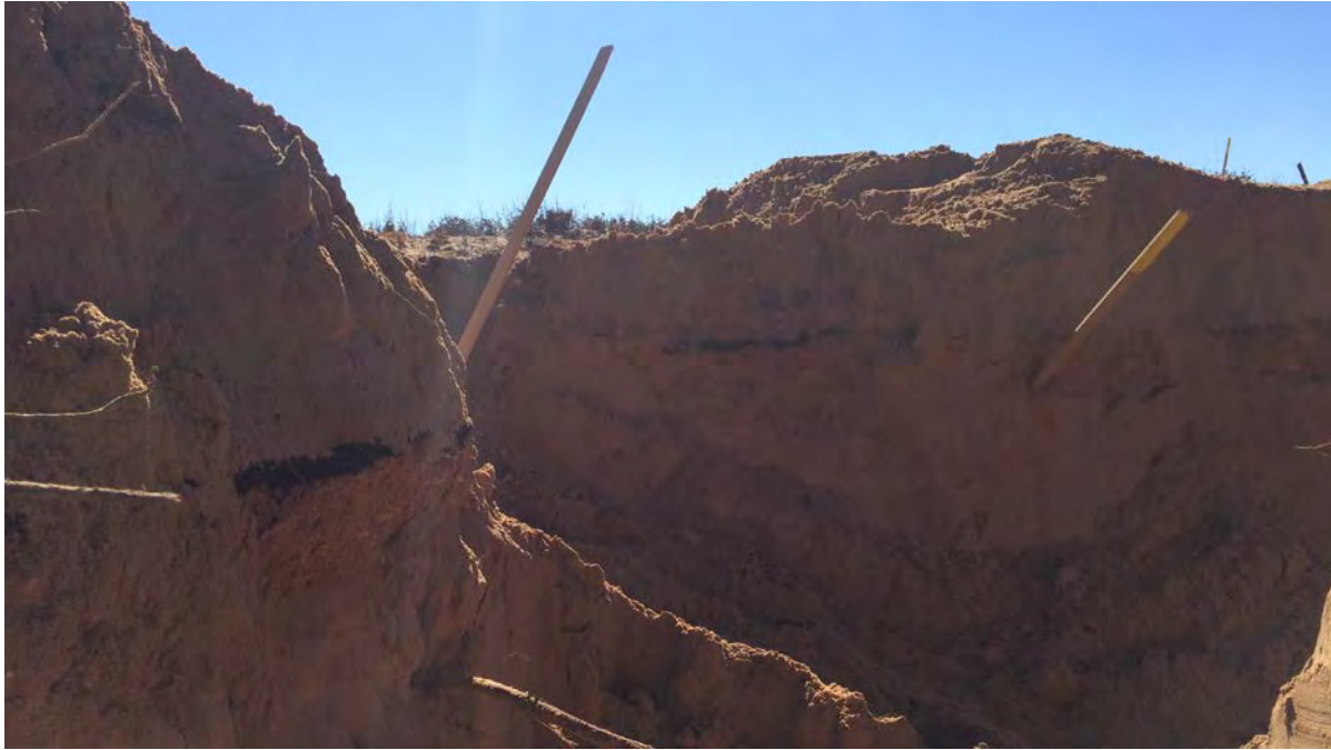
Figure 1 – In accordance with the workplan, we first excavated several trenches to clearly define the extent of visible hydrocarbon staining. In this image, the staining is clear above the former caliche pad. The oil and pad were covered with sand after the spill to prevent any impact to cattle.
