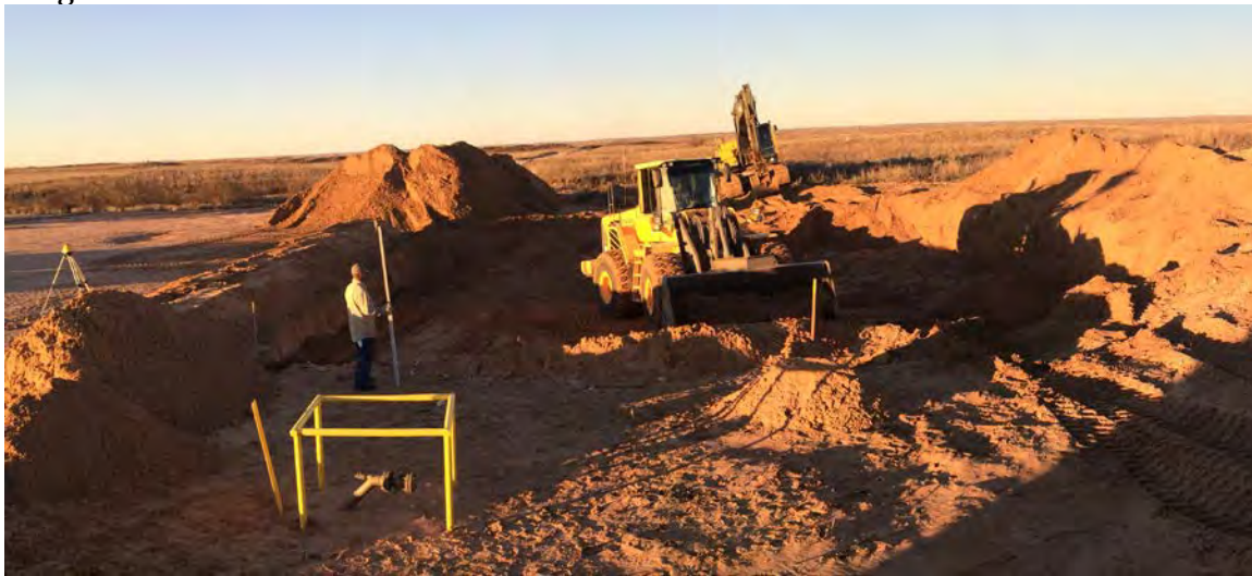
Figure 5 – The last load of suspected salt-impacted soil is placed on the level remediation cell
