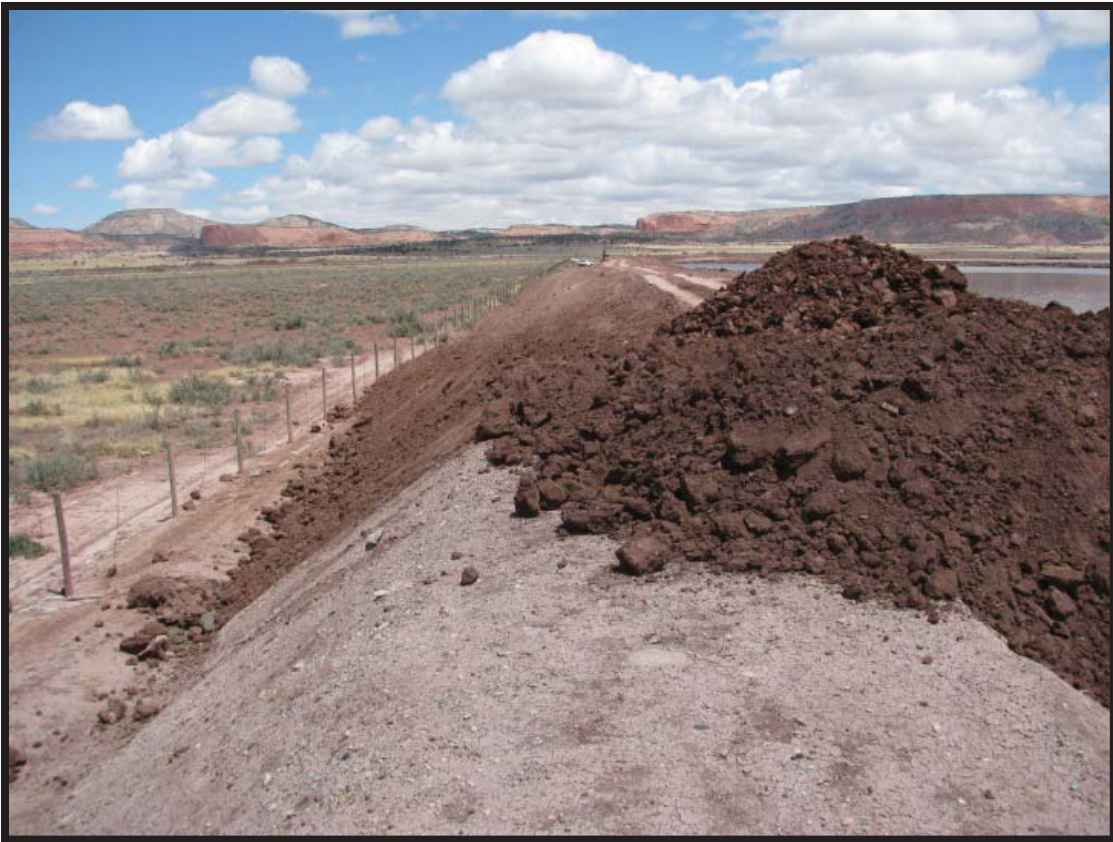
Photo #3: Pond 7/8 West Berm Under Construction - Looking North (Note how the new crest alignment is shifted to the east)
