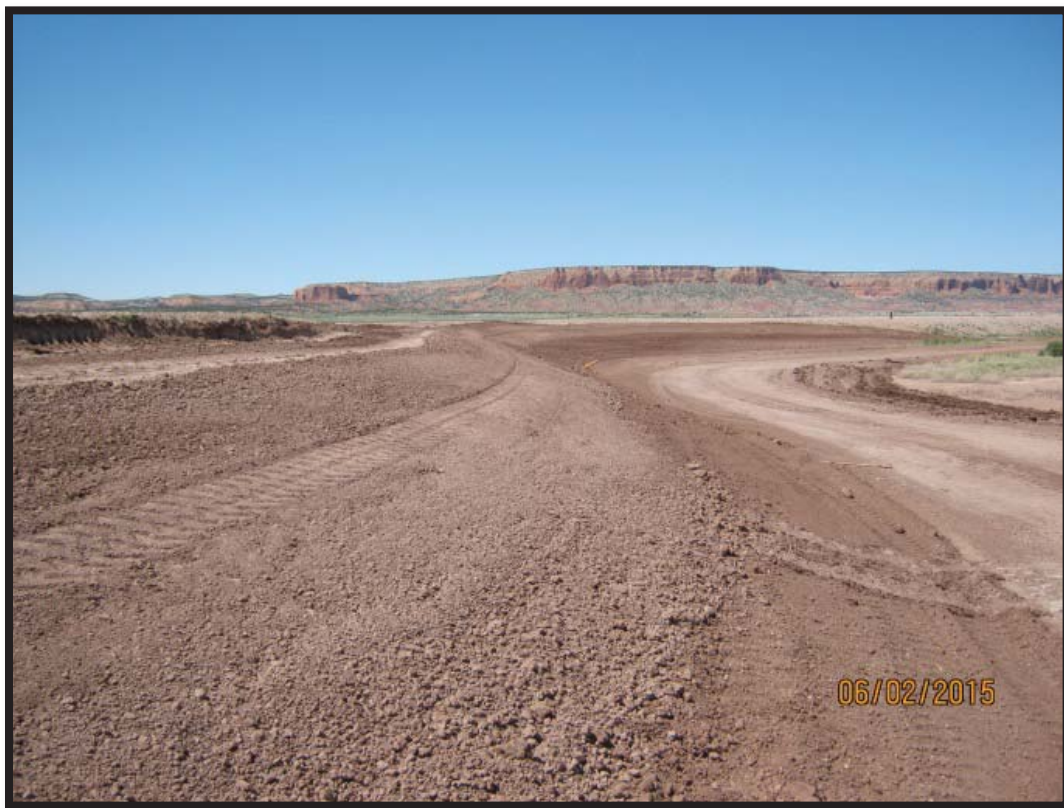
Photo #12: Pond 7/8 and Pond 11 South Berms Under Construction, Nearly Complete - Looking Northeast
