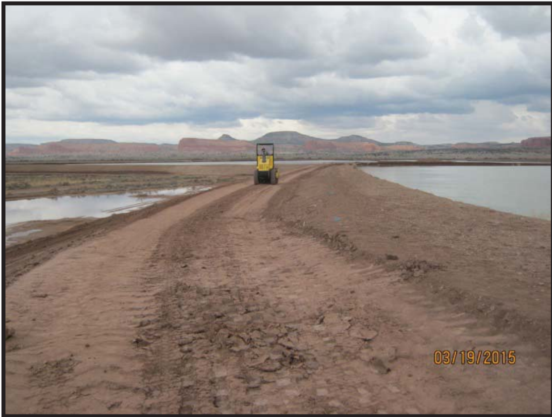
Photo #9: Pond 6 West Berm Under Construction, Nearly Complete - Looking North
