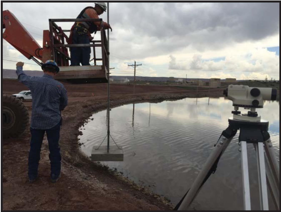
Photo #1: Installation of a Staff Gauge in Pond 9 - Looking East
