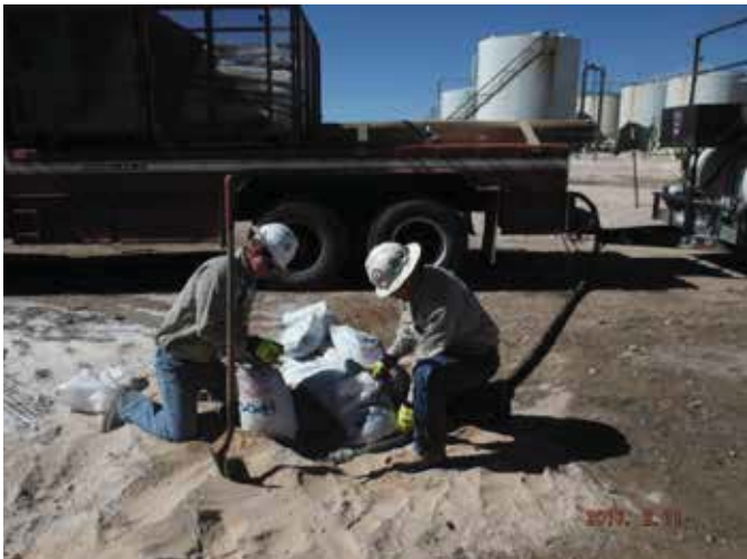
Plugging soil bore #2, facing west 2/11/16
