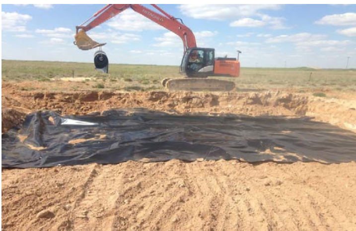
View of liner placement in excavation, facing north.
