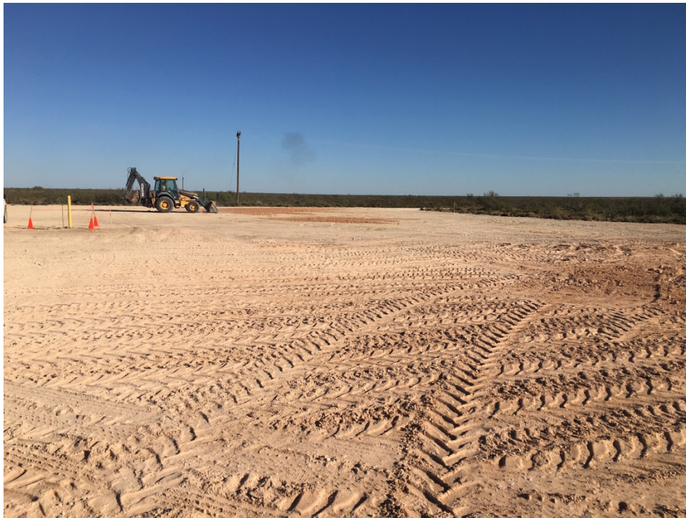
Photo 7 - View of Site during wheel compacting and grading facing northwest
