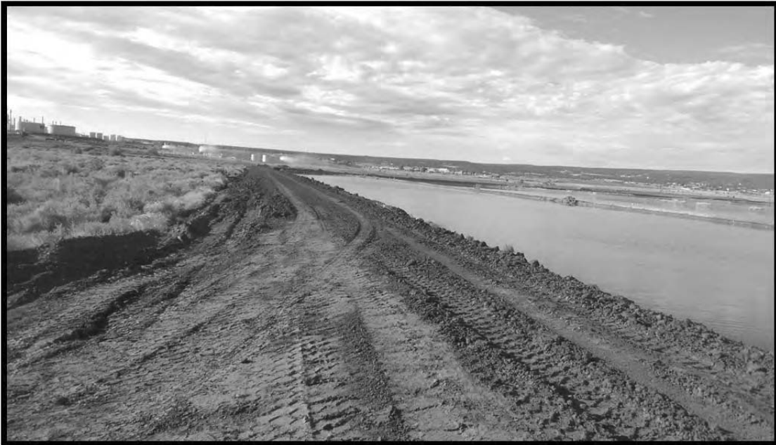
Photo #18: Pond 11-12 Berm Fill Repair Completed.
