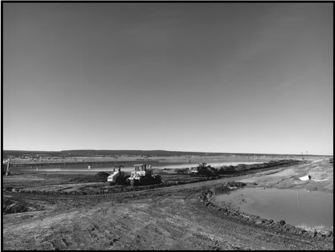
Photo #19: Pond 9 Start of Fill Placement on North Berm
