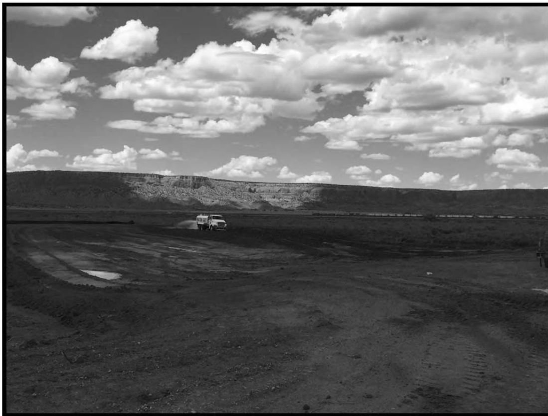
Photo #14: Moisture conditioning soil in the borrow area.
