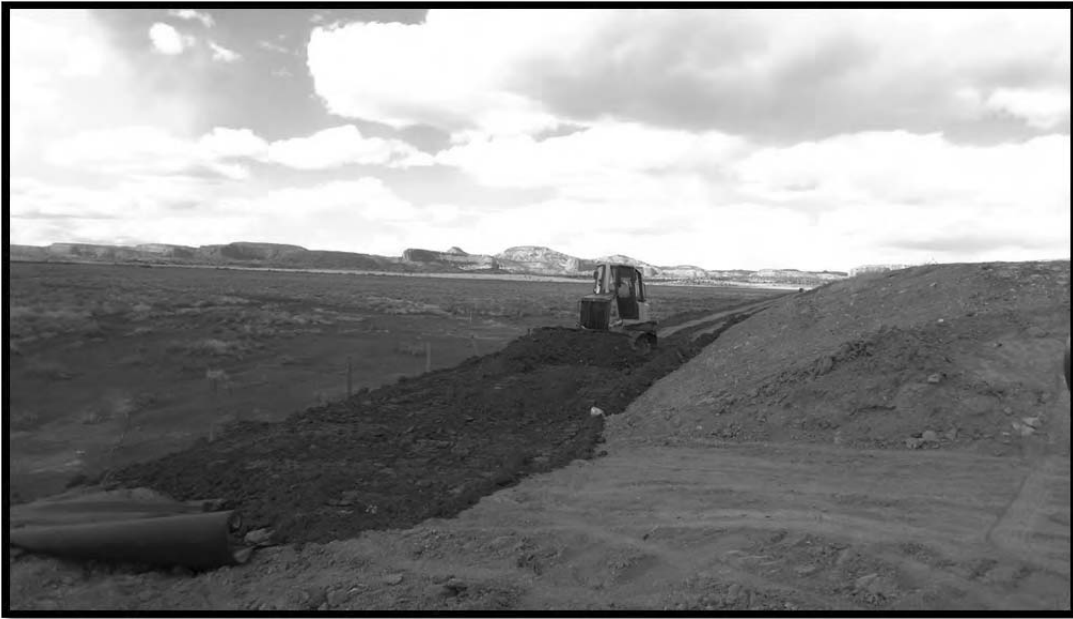
Photo #15: Pond 7/8 West Berm Fill Over Geotextile
