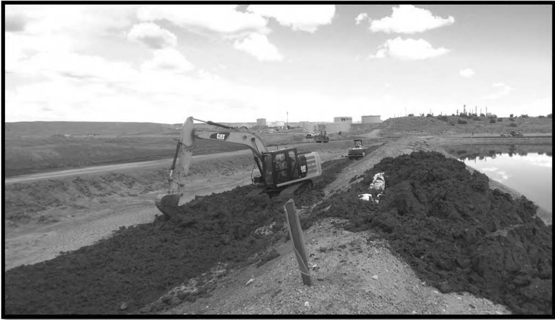
Photo #21: Pond 9 Start of Fill Placement on North Berm Removing Base Material and Placing it on the Interior
