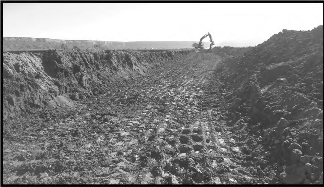
Photo #17: Pond 11-12 Berm Being Removed and Reworked
