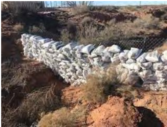
Installing bags for erosion control
