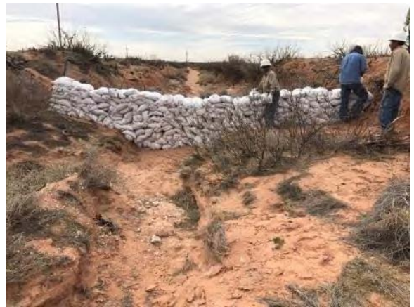
Installing bags for erosion control
