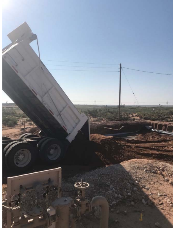
Backfilling with imported soil
