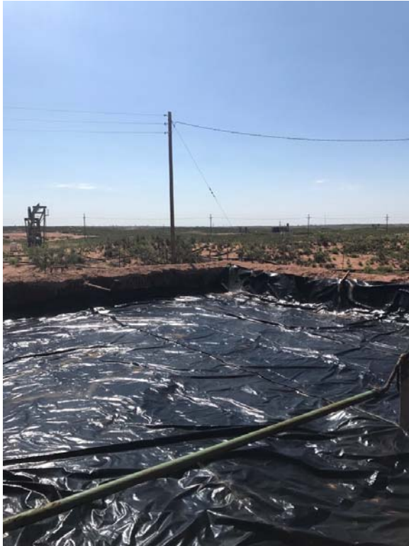
Installed 20-mil, reinforced poly liner
