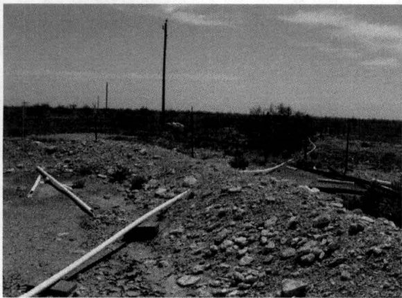
Berm area lacks liner system- awaiting construction w/ liner system
