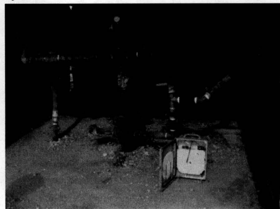
Wellhead with chart recorder, but pressure is only at 200 psig. Well needs recharging for MIT tomorrow.
