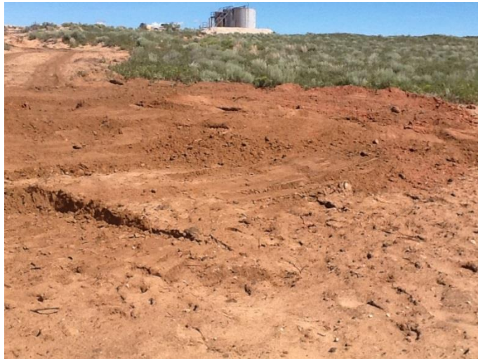
Backfilled Test Trench Area to Grade
