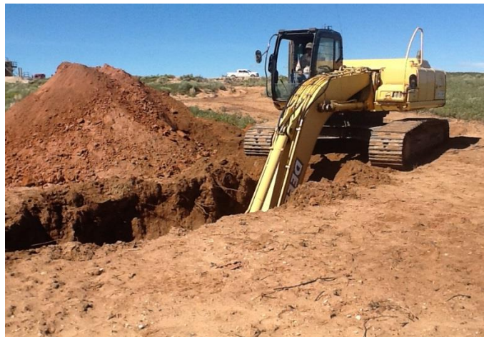
Backhoe reaches capacity at 18.5' bgs
