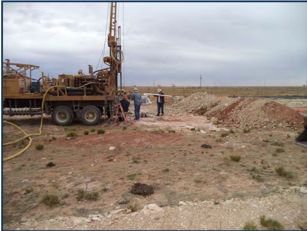
Photograph #5: View of monitoring well MW-1 installation with soil remaining on liner being stockpiled for eventual disposal.
