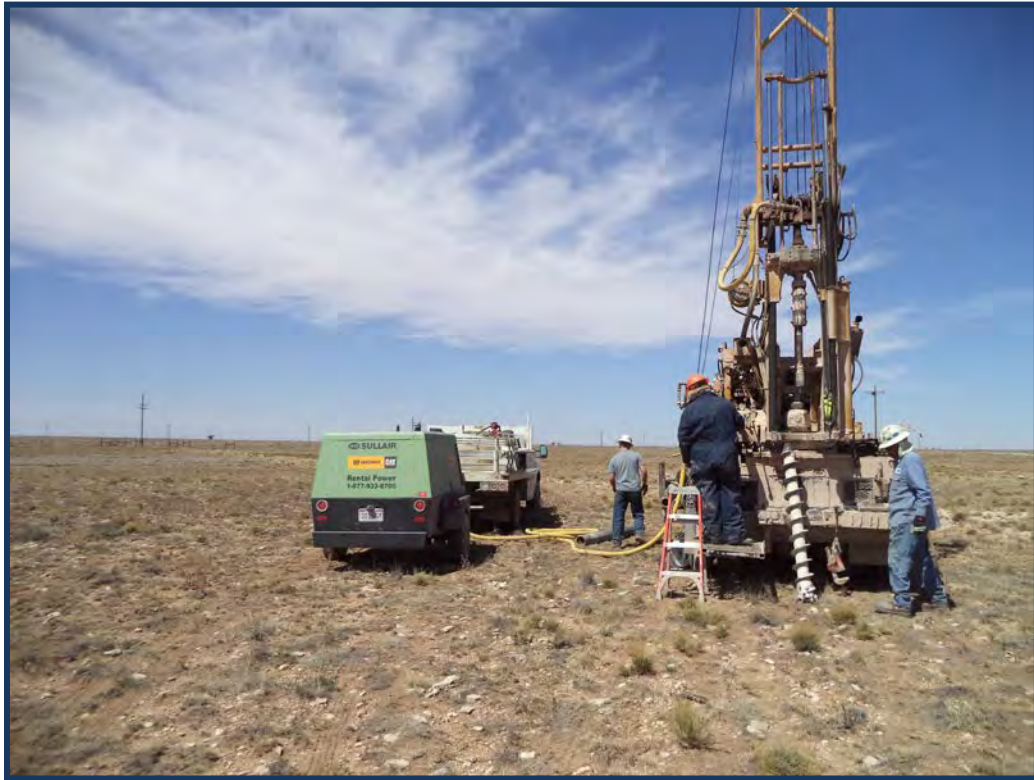
Photograph #9: View of drilling rig set-up on monitoring well MW-3.
