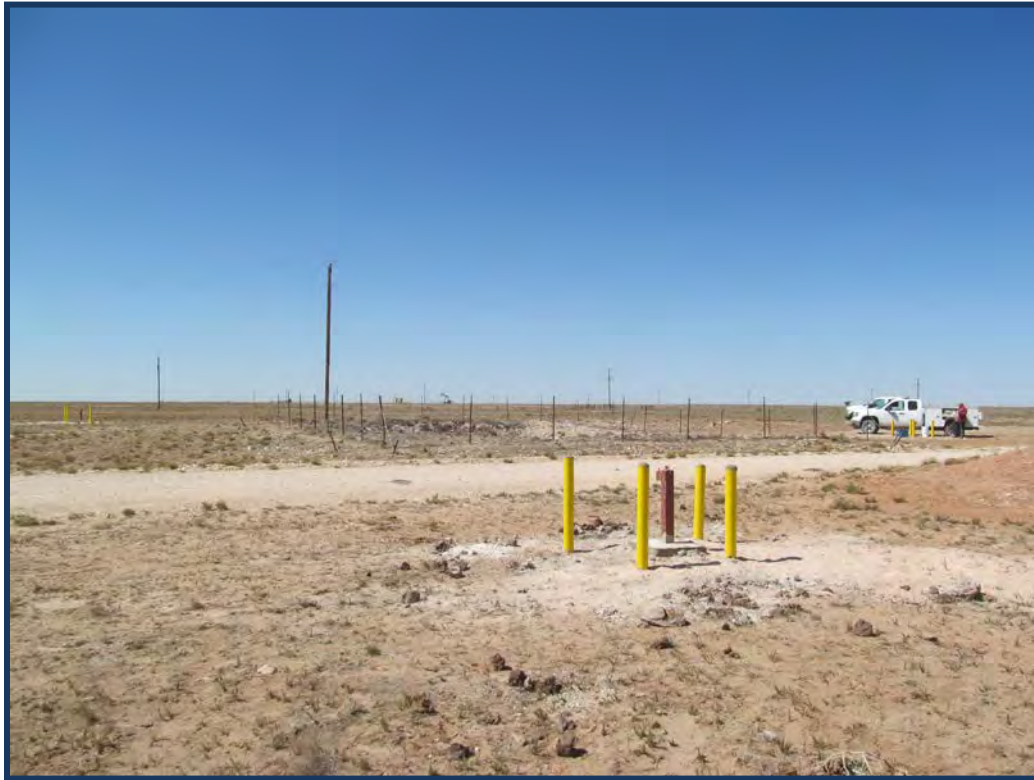
Photograph #17: View of monitoring well MW-2 surface completion (typical).
