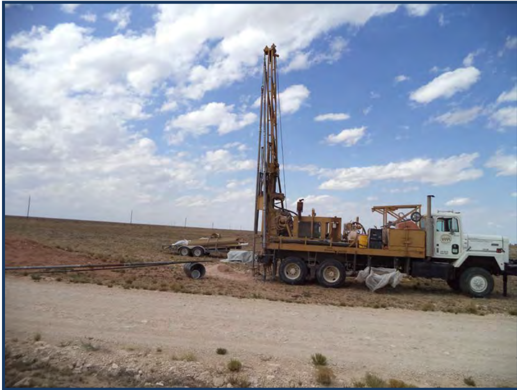
Photograph #7: View of monitoring well MW-2 drilling.
