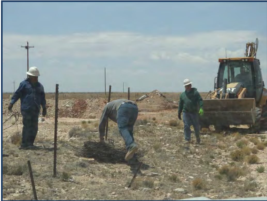
Photograph #13: Removal of existing fence, plastic liner and contaminated soil stockpiled for eventual removal in background.
