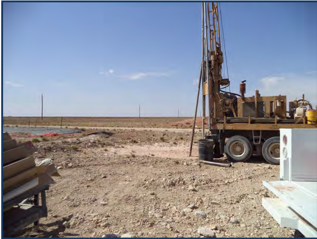
Photograph #3: View of monitoring well MW-1 drilling.
