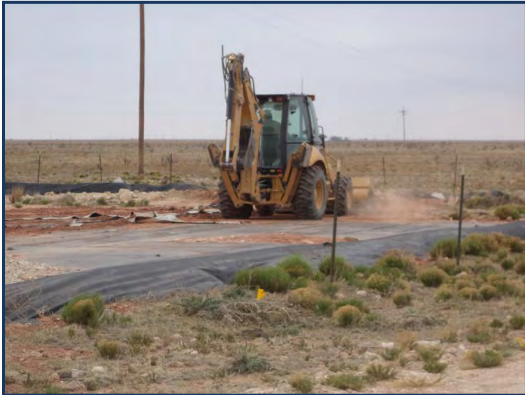
Photograph #11: View of cleanup of contaminated soil previously stockpiled on plastic liner.
