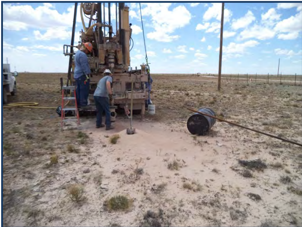
Photograph #10: View of monitoring well MW-3 drilling.
