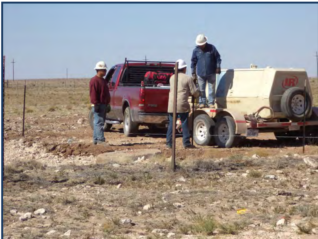
Photograph #14: Air compressor used for installation of T-Posts in rocky terrain.
