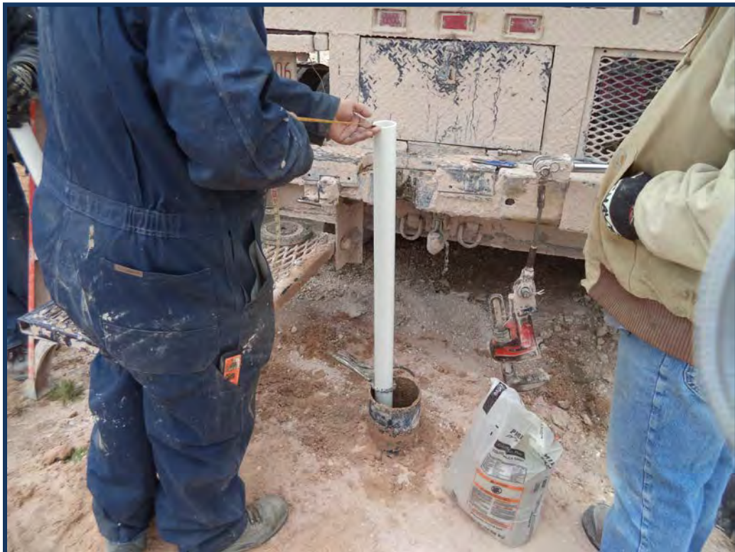
Photograph #6: Additional view of monitoring well MW-1 installation.
