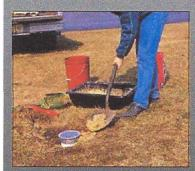
The hole and pipe are carefully back-filled with sand. The top 12 inches (300 mm) of the hole (OUTSIDE of the PVC Pipe) are back-filled with concrete,
