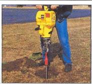
The rod monument is driven into the ground, a section at a time, to refusal\*. The top of the last rod should be about 6 inches (150 mm) below the surface, \*See page 15
