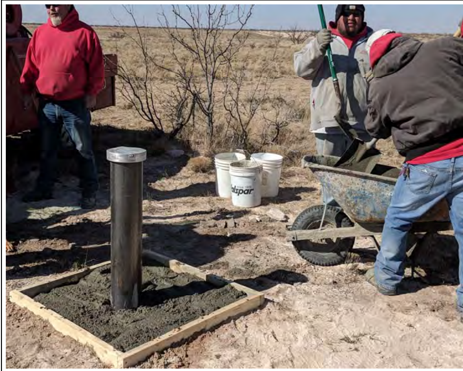
7. Monitor well DBS-10: Peterson constructing the well pad.
