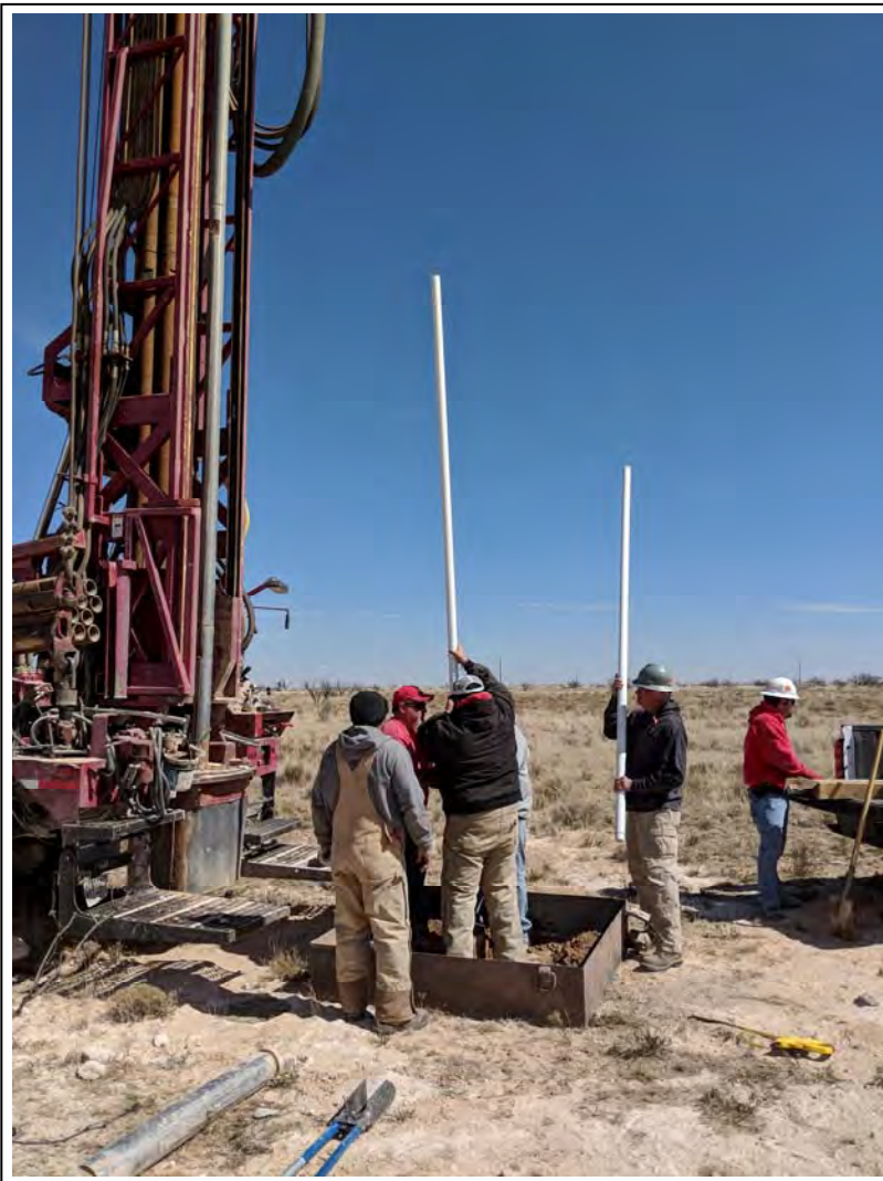
5. Monitor well DBS-10: Peterson suspending and assembling 2-inch-diameter SCH 40 PVC well casing.
