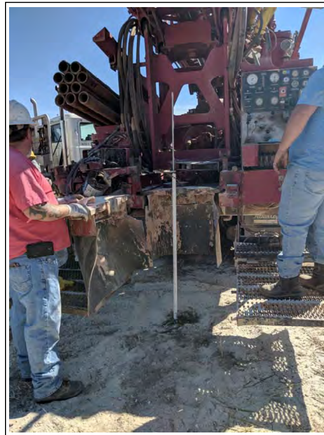
2. Installation of survey monument SMP-3. The monument was centered and suspended within the borehole, and the anchor plate and sleeve were carefully placed before installing cement grout to anchor the monument in sandstone.
