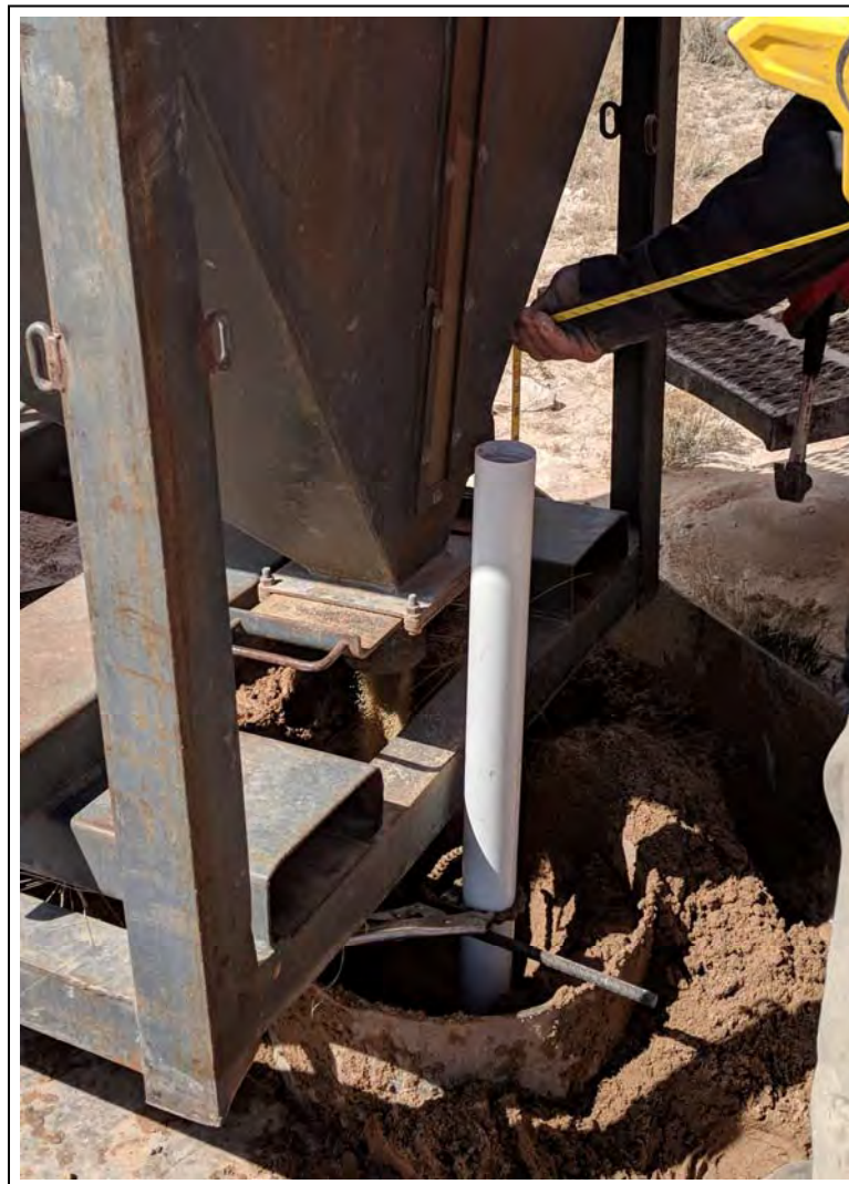
6. Monitor well DBS-10: silica sand being poured down the borehole, extending from bottom of borehole to approximately 5 feet above the top of well screen. Bentonite chips were then placed on top of the silica sand filter pack, extending to depth of 15 feet bgs. Cement grout was then used to fill the remainder of the annulus.
