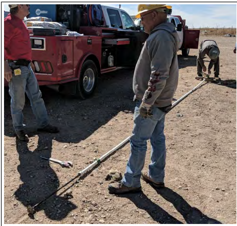
1. Peterson assembling a survey monument consisting of a stainless steel rod inside a PVC sleeve. The crew greased the inside of the sleeve to allow the rod to move freely within the sleeve.
