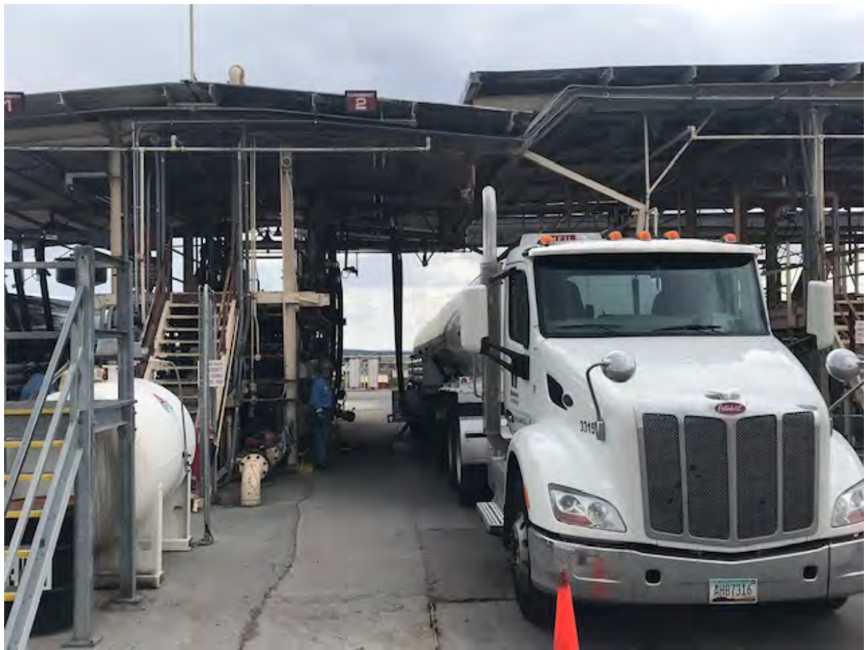
Photo 9 – Looking west at loading bay 2.
