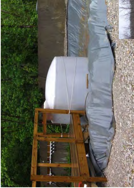
SO4 Feed Tank 15% Epson Salt & 100 mg/l NH4
