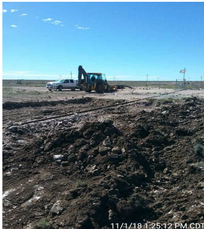
View Southwest– Area of NWS-1 and WSW-1
