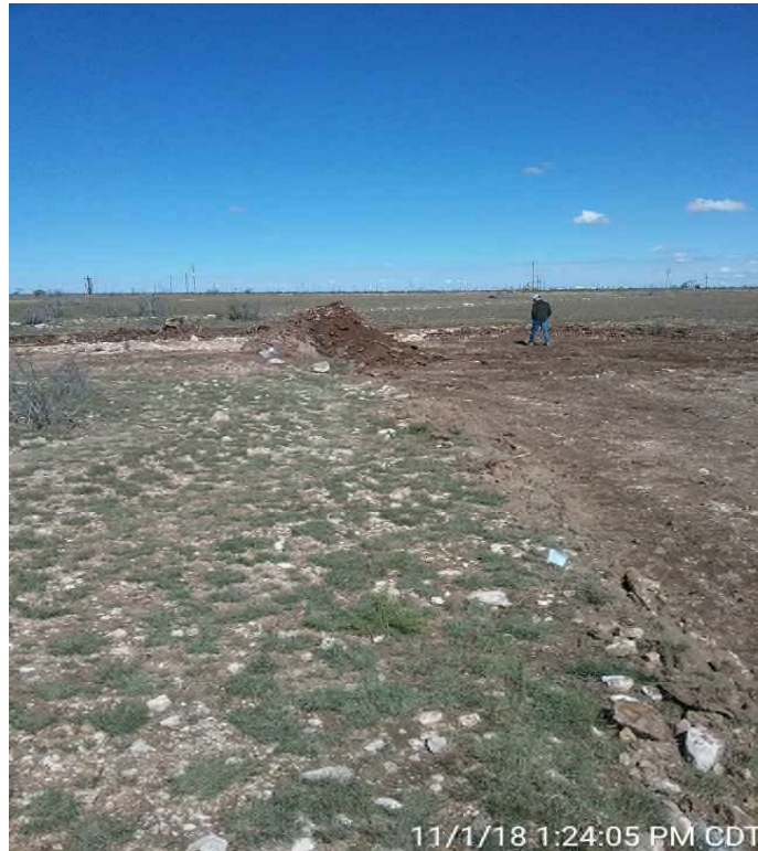
View Northeast– Area of WSW-1 and WSW-2
