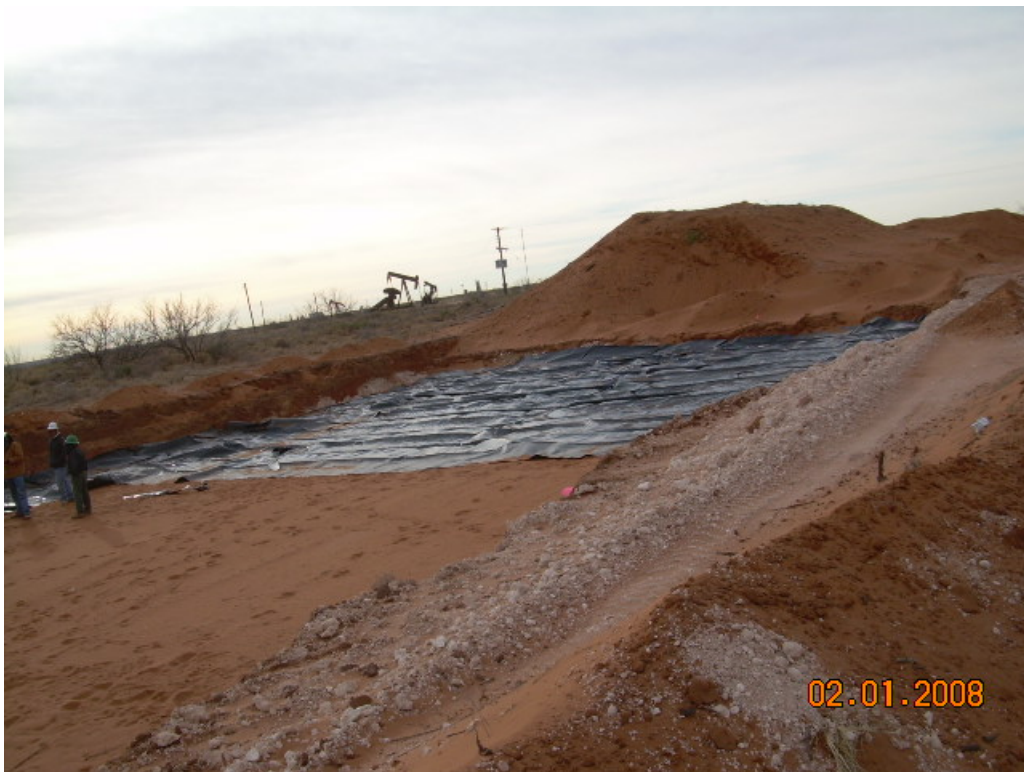
Photograph No. 10 – Installation of 40-mil liner over central deep excavation.
