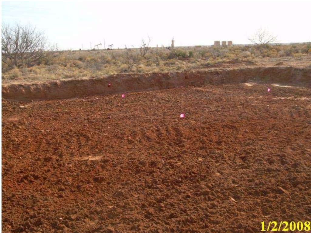
Photograph No. 5 – Looking easterly across excavation.
