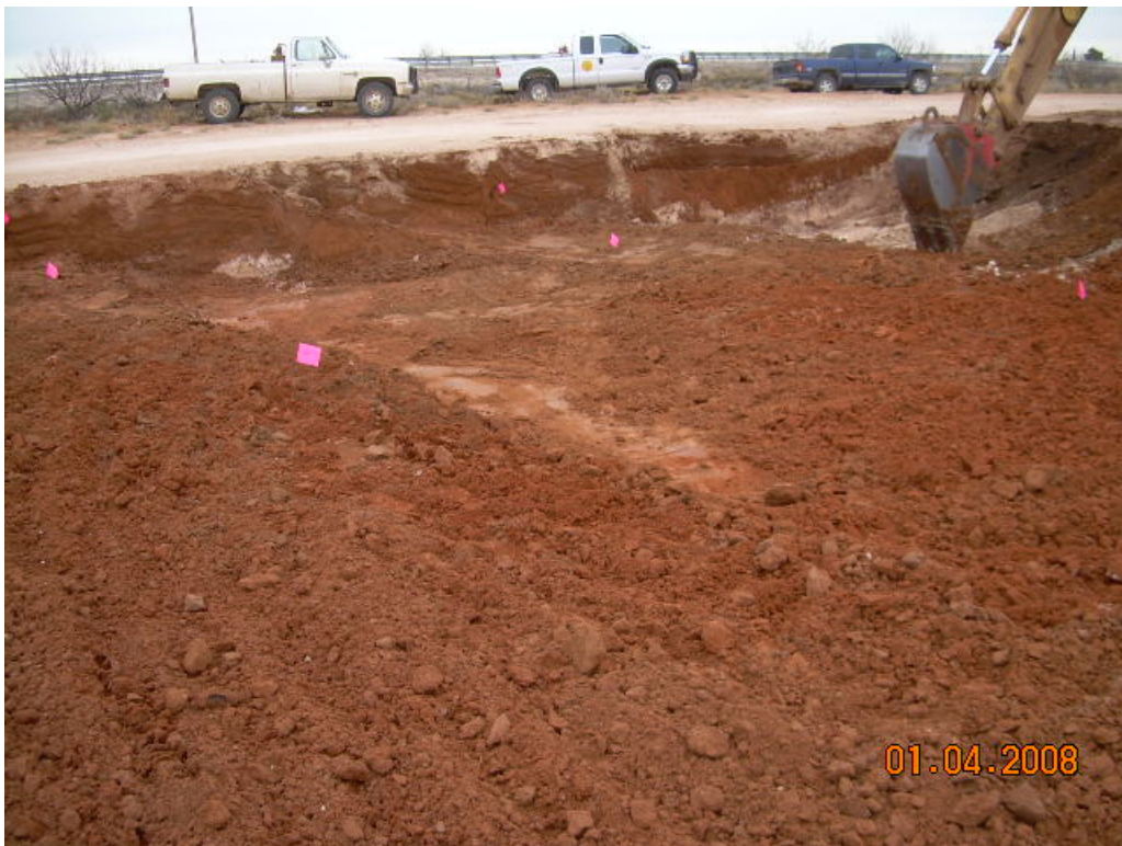
Photograph No. 6 – Looking west across excavation.
