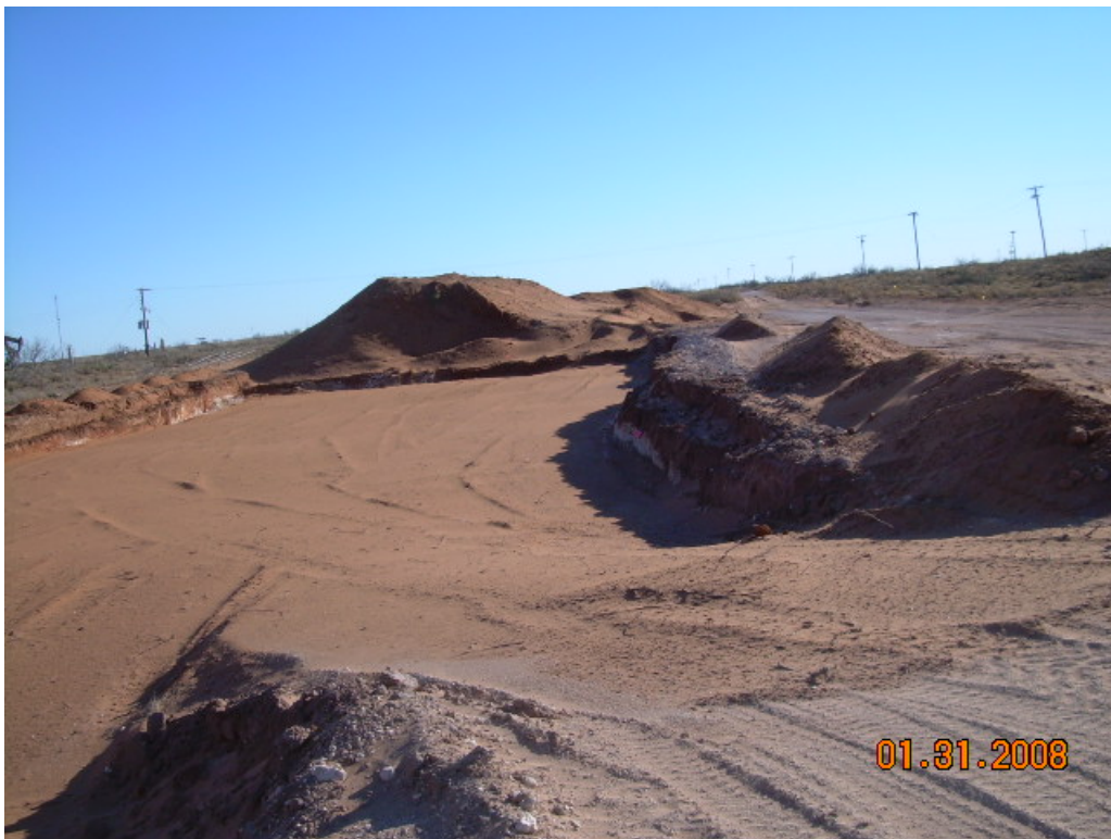
Photograph No. 8 – Looking southerly across excavation prepped for liner.
