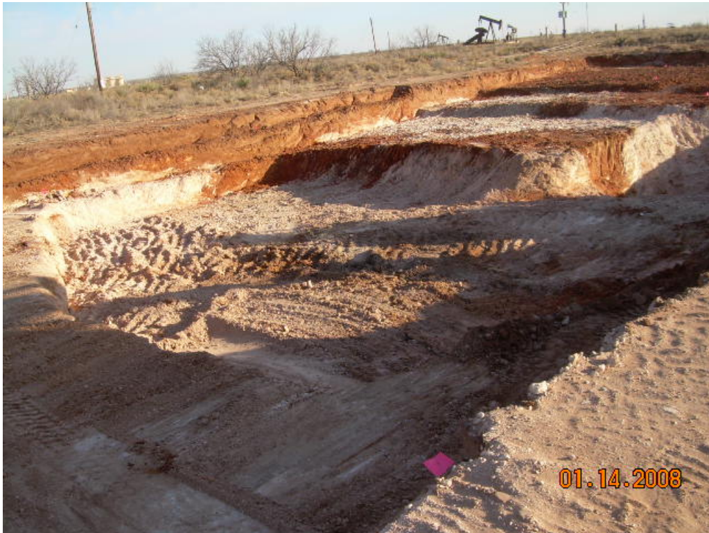
Photograph No. 7 – Looking easterly across excavation.
