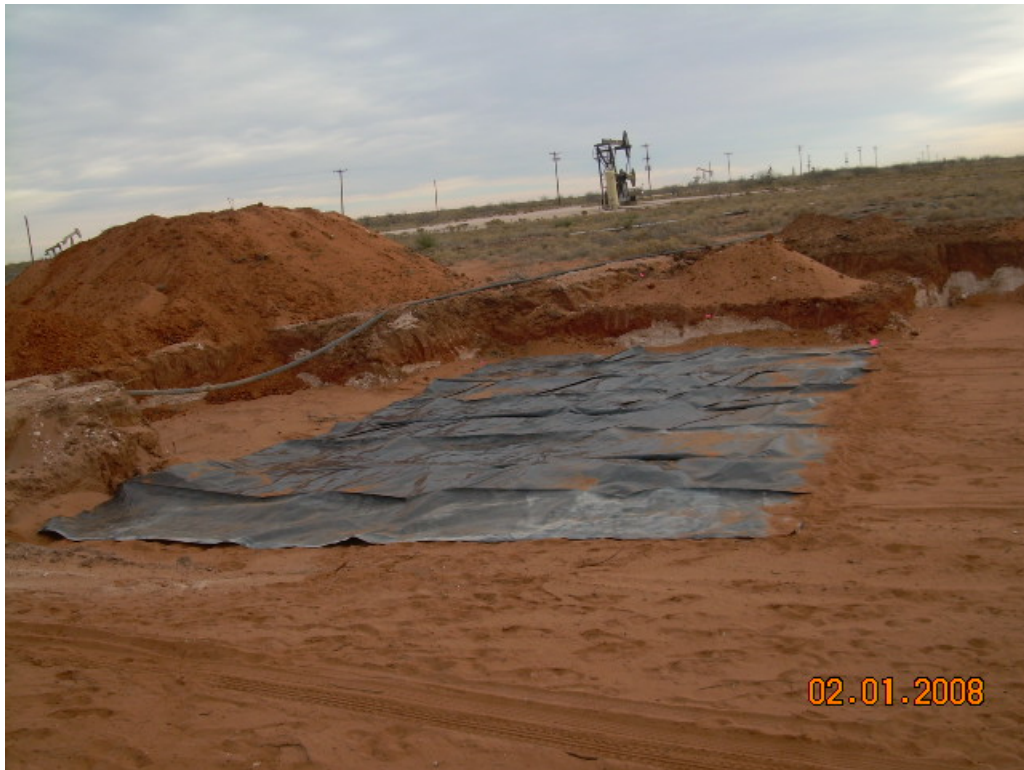
Photograph No. 9 – Installation of 40-mil liner over northern deep excavation.
