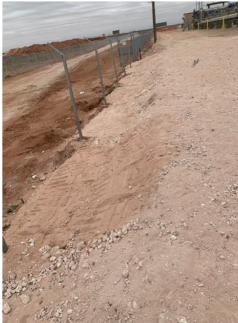
Backfilled Excavation – Facing North
