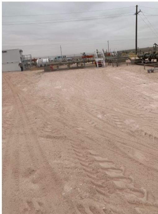
Backfilled Excavation – Facing South
