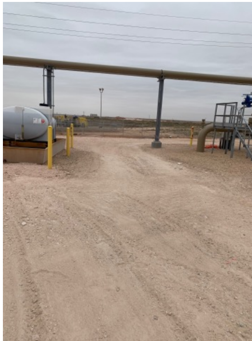
Backfilled Excavation – Facing West
