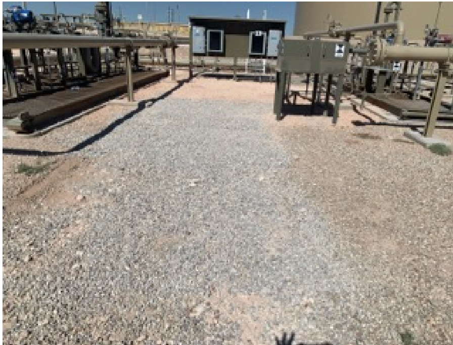
Backfilled Excavation – Facing North
