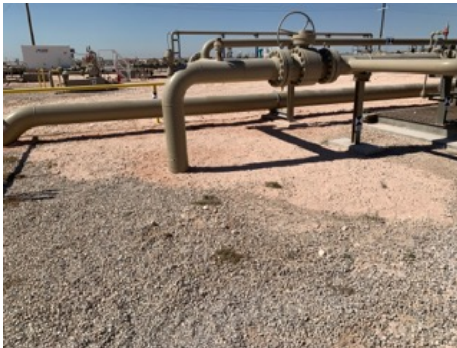
Backfilled Excavation – Facing West
