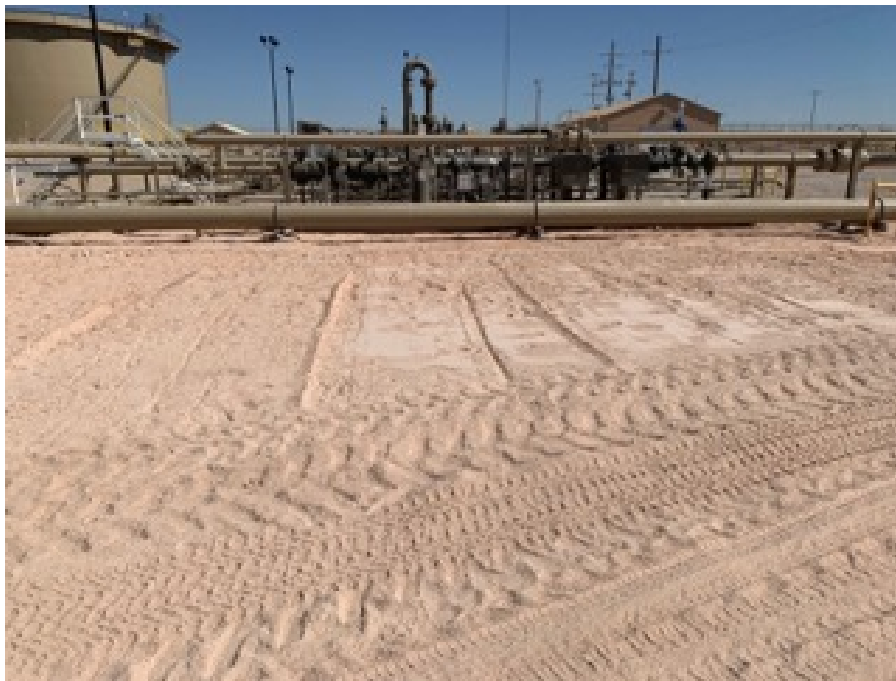
Backfilled Excavation – Facing East
