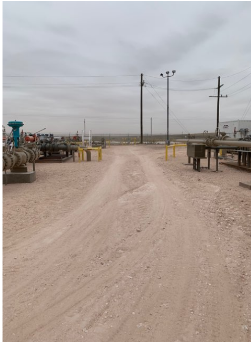
Backfilled Excavation – Facing South
