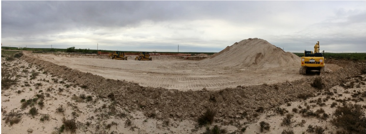
Figure 3: Photograph of containment berm along southern half of northern portion of release area. Containment berm was constructed during the initial response on June 3rd. Photograph is the day R.T. Hicks Consultants took over remedial activities on June 10th. Date/Time: 2019-06-10 17:51:14. GPS: 32.4440167 N, 103.5732583 W.
