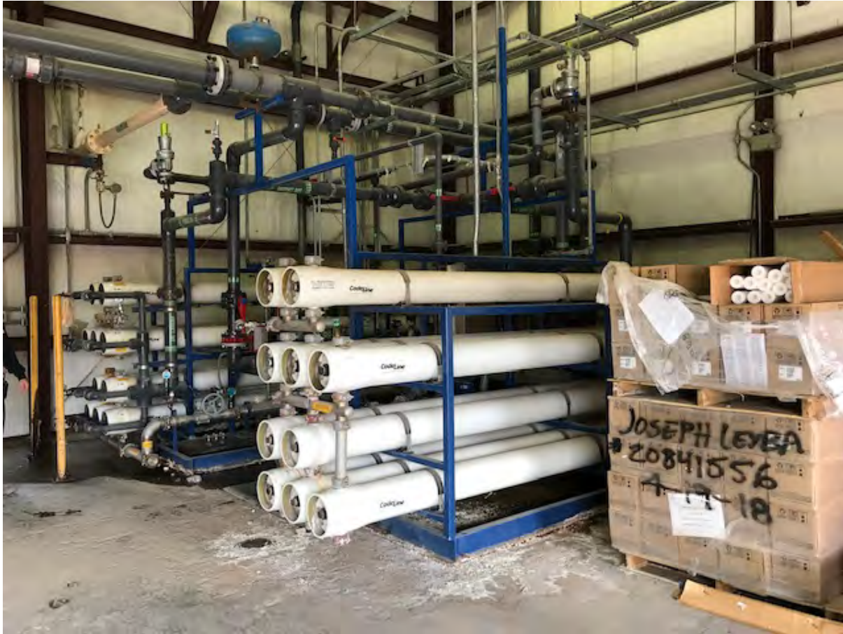
Step 2: Reverse Osmosis water softening system.
