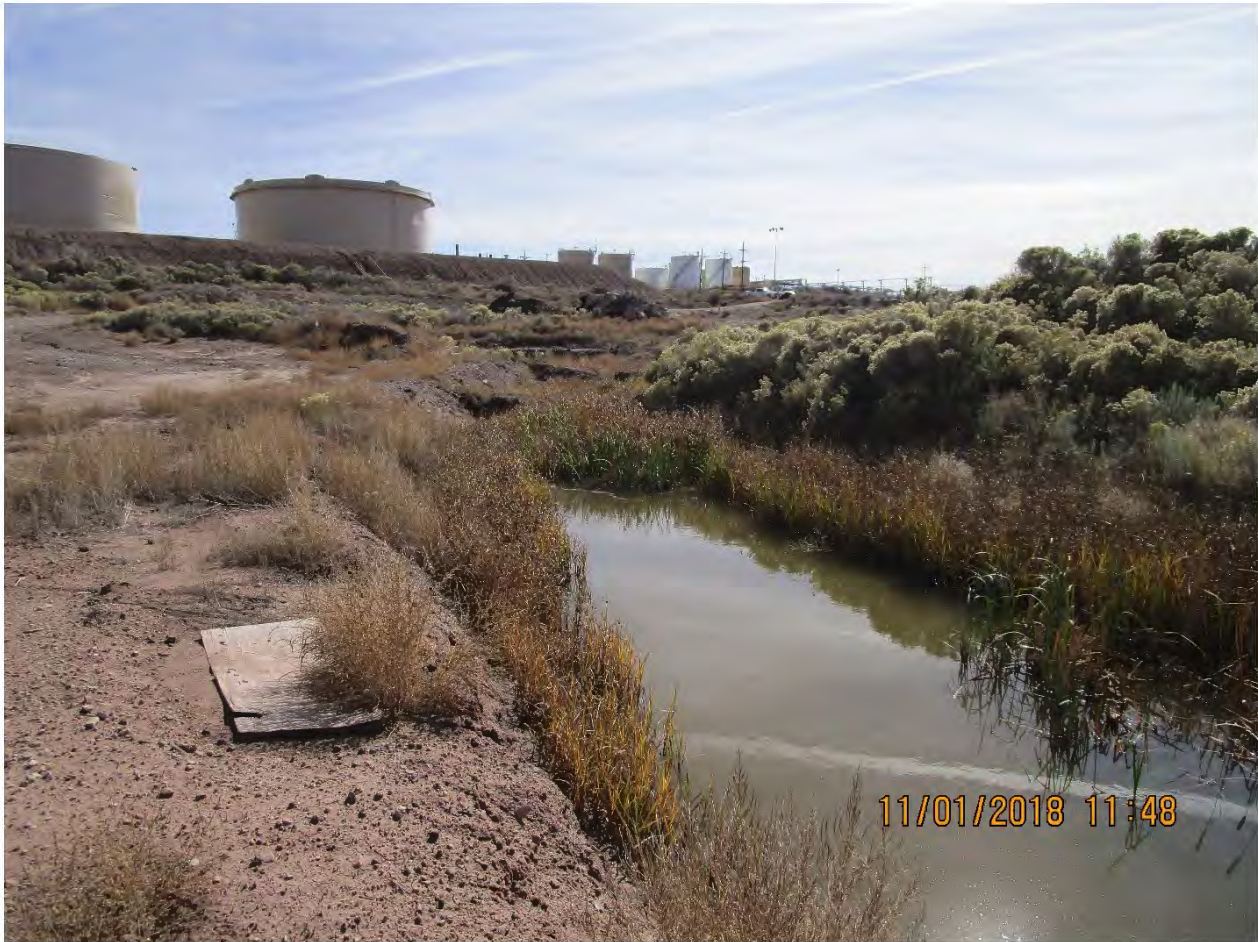
Photo No. 1 of lowermost (northern) end of retention ditch. Oil stained vegetation shown around edges of ditch but no recoverable product on water.
