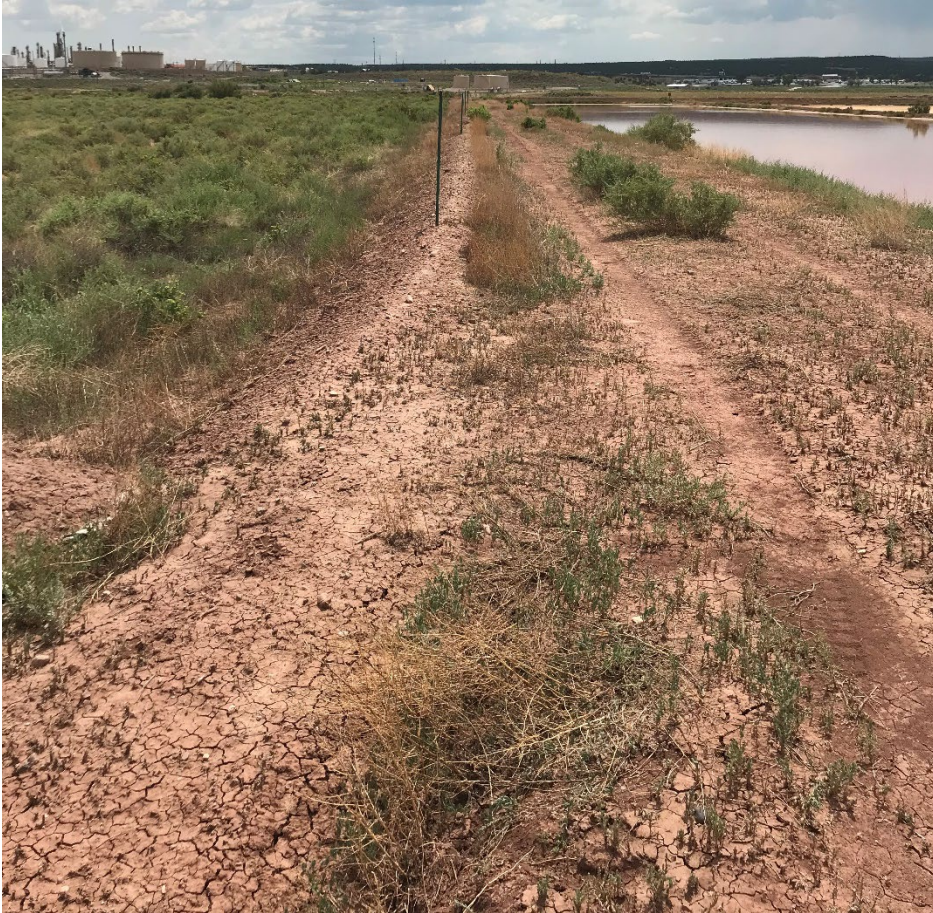
Figure 7: North Cell: Looking South along west wall
