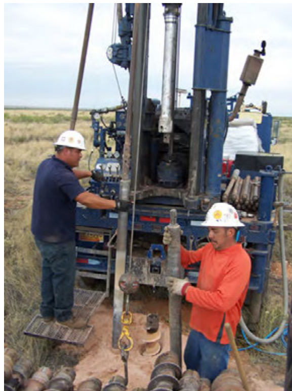
Photograph 2. HSA drilling and continuous core sampling CH-1. Driller and helper each holding 5-foot long sampler.
