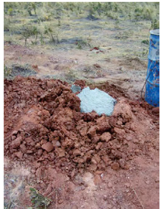
Photograph 36. Typical borehole plugged to surface.
