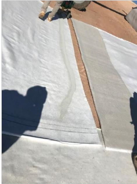
11-13-18 Free bentonite applied to GCL seams.
