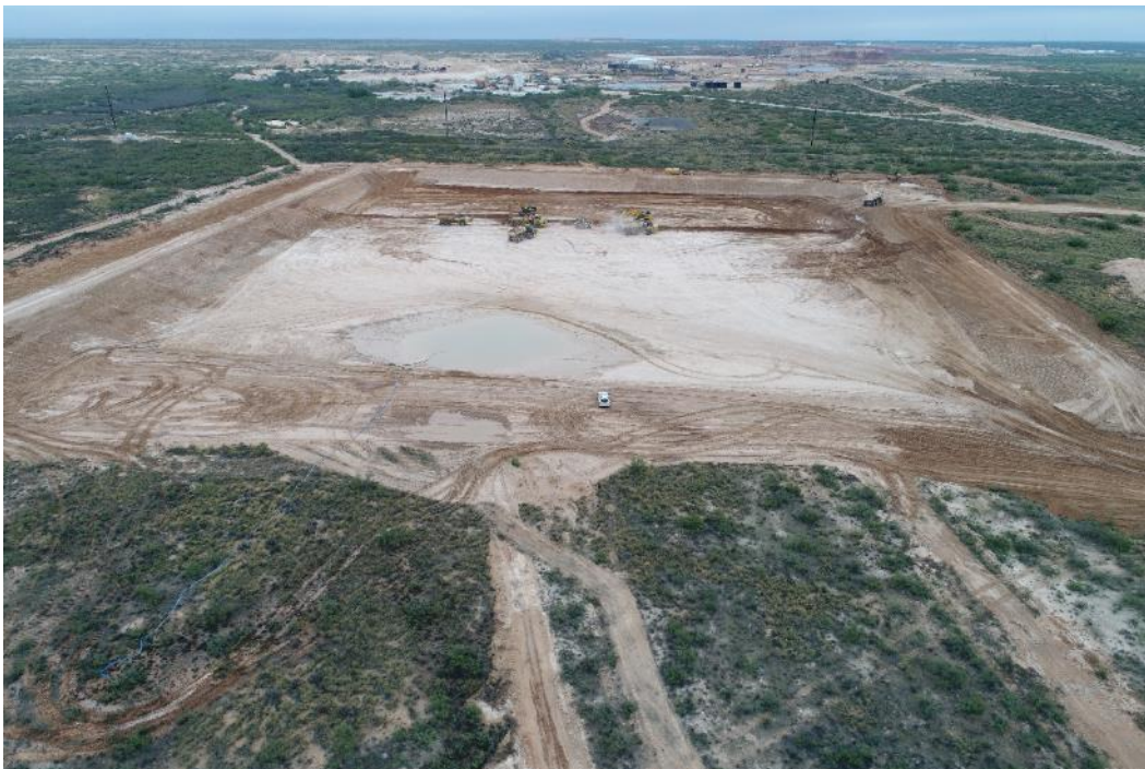
10-23-18 Excavation and berm construction from above. East view.
