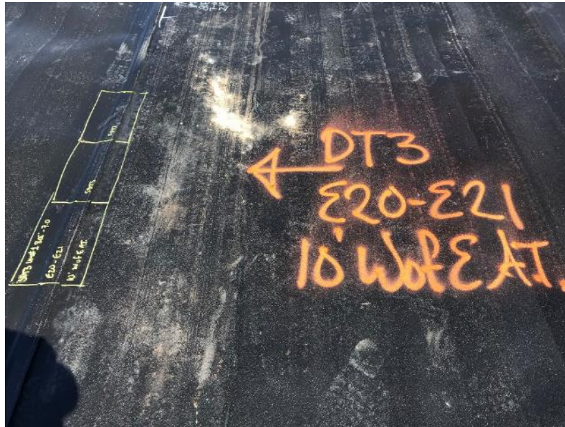
11-13-18 Textured FML panel marked with a destructive test to be cut.
