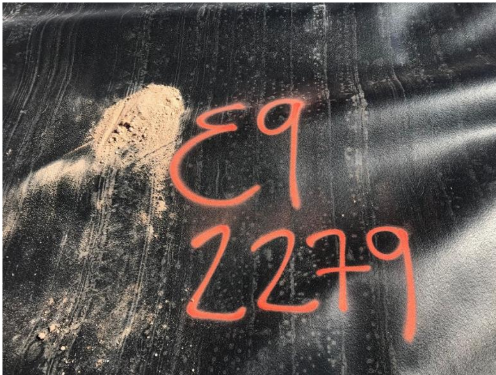
11-13-18 Textured FML panel installed and marked with panel number and roll number.
