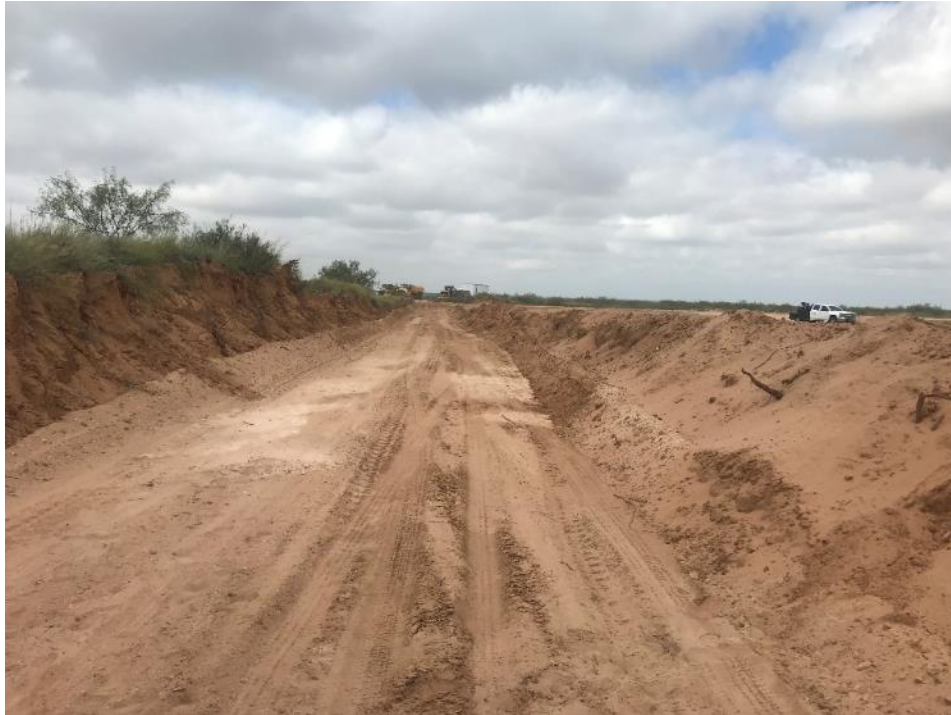
9-23-18 Area of deep roots cleared. West view.
