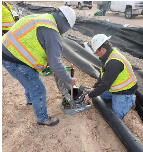
1-08-19 Fusing of HDPE pipe for Leachate Collection System. Note geotextile and bedding aggregate.
