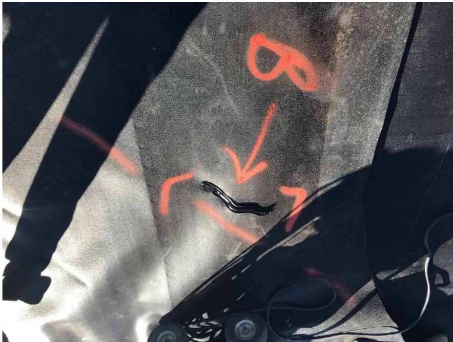
11-14-18 Bead repair on installed FML.
