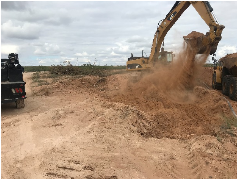
9-17-18 Clear and Grub of project area. Northwest view.
