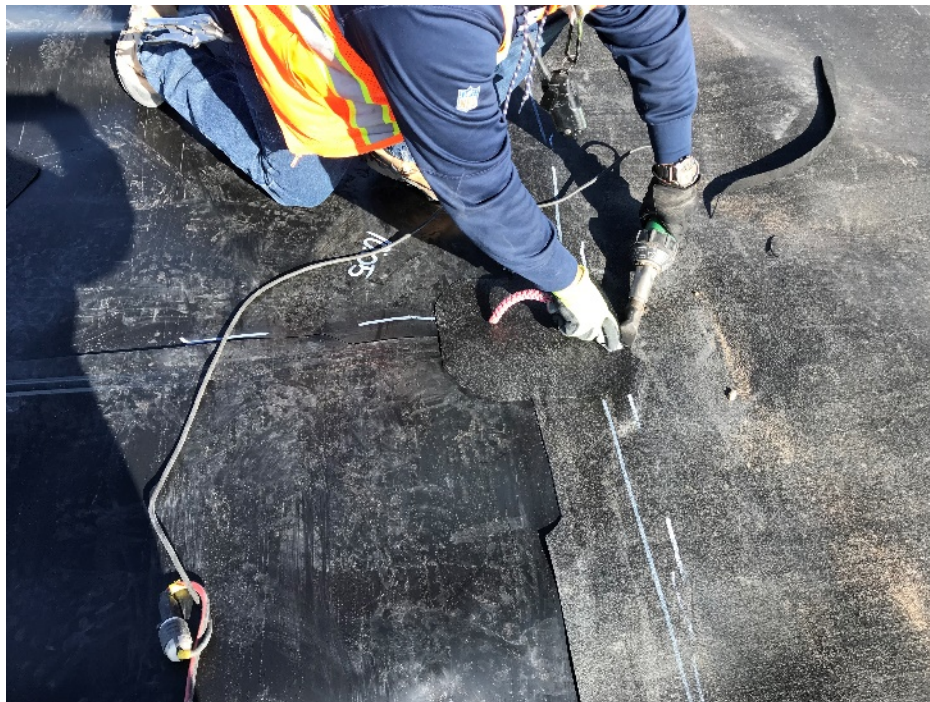
11-20-18 Patch repair in progress, primary liner.
