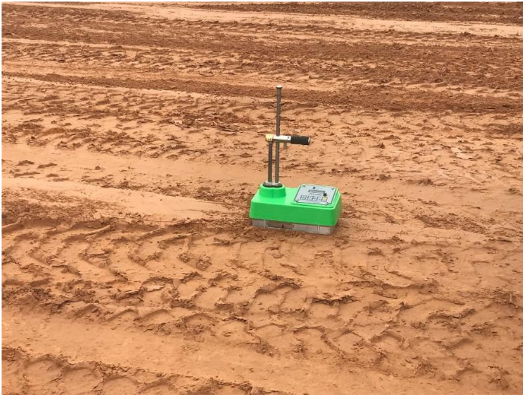
10-31-18 Berm construction density test in progress.
