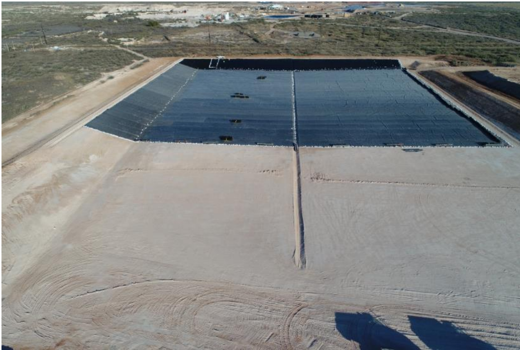
11-19-18 FML liner progression from east to west. East view.
