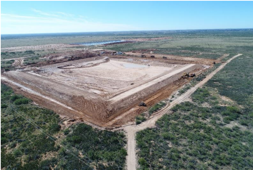
10-25-18 Landfill excavation, berm and perimeter drainage construction. Southwest view.
