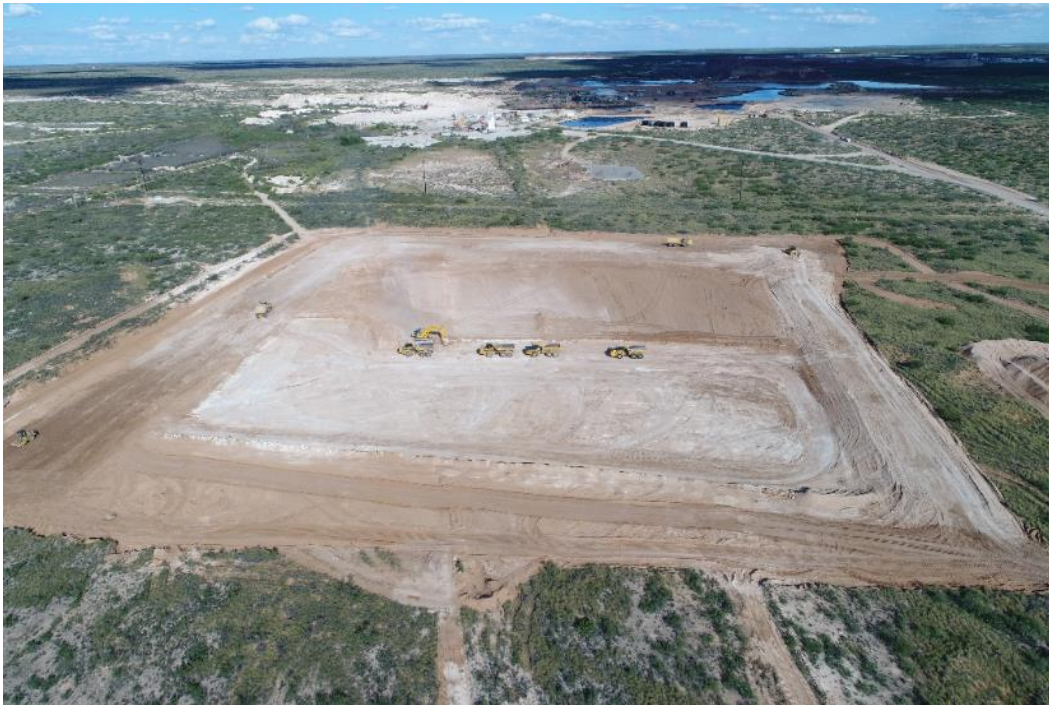
10-9-18 Excavation and berm construction from above. East view.
