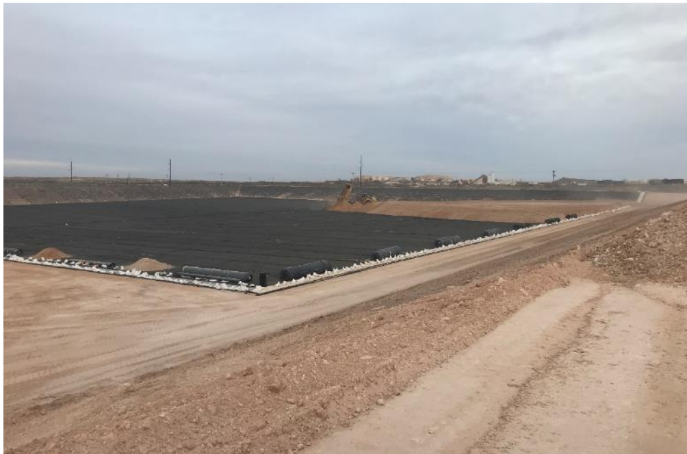
12-5-18 Protective Soil Layer installation in progress. Northeast view.
