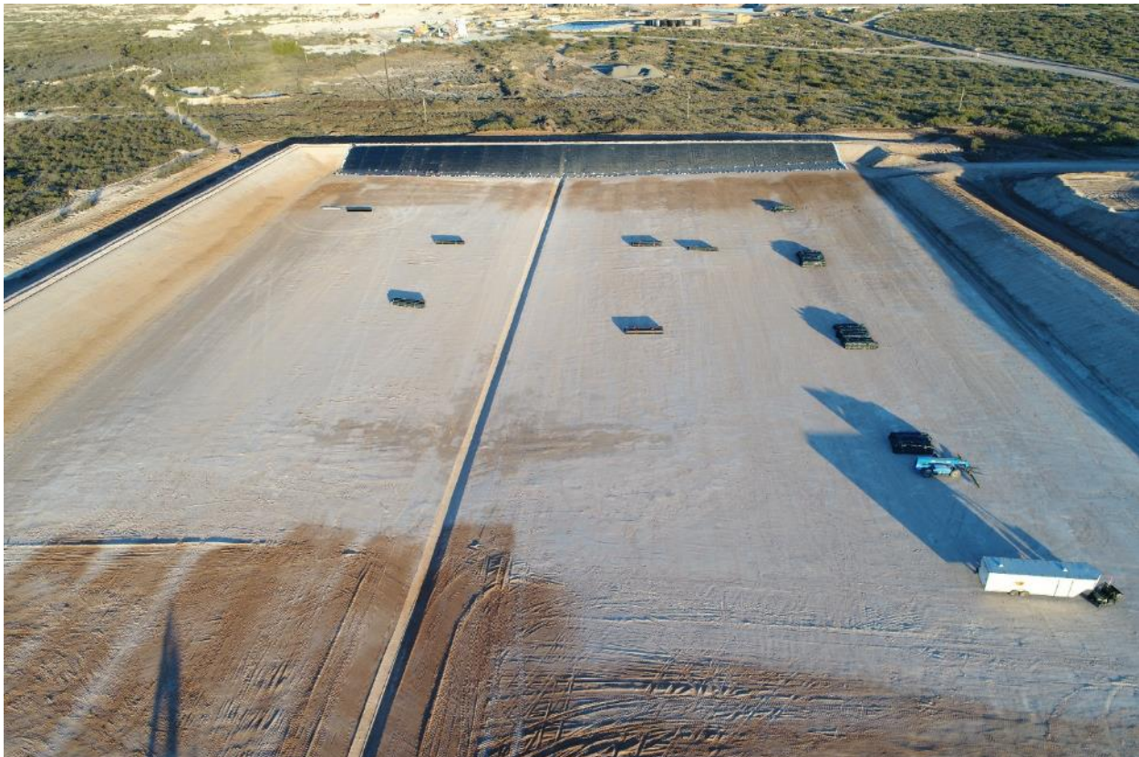
11-13-18 Textured FML secondary liner installed on the east slope. East view.
