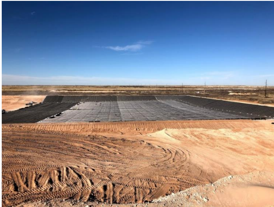
11-28-18 Liner installation progression. North view.
