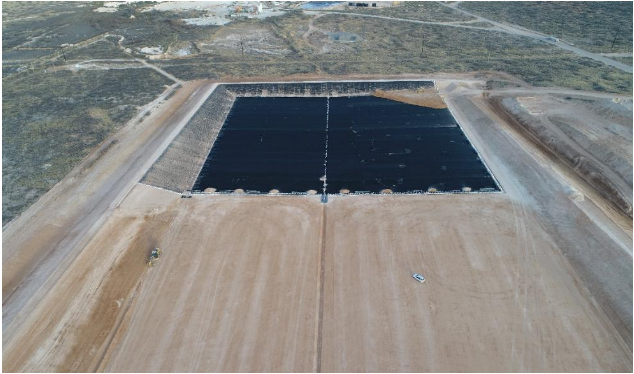
12-4-18 Completed geosynthetics installation of Cell 1A. Protective Soil Layer placement in southeast corner. Note Cell 1B excavation progression. East view.
