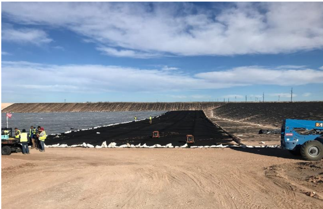
12-1-18 Installation of single-sided geocomposite on cell floor. North view.
