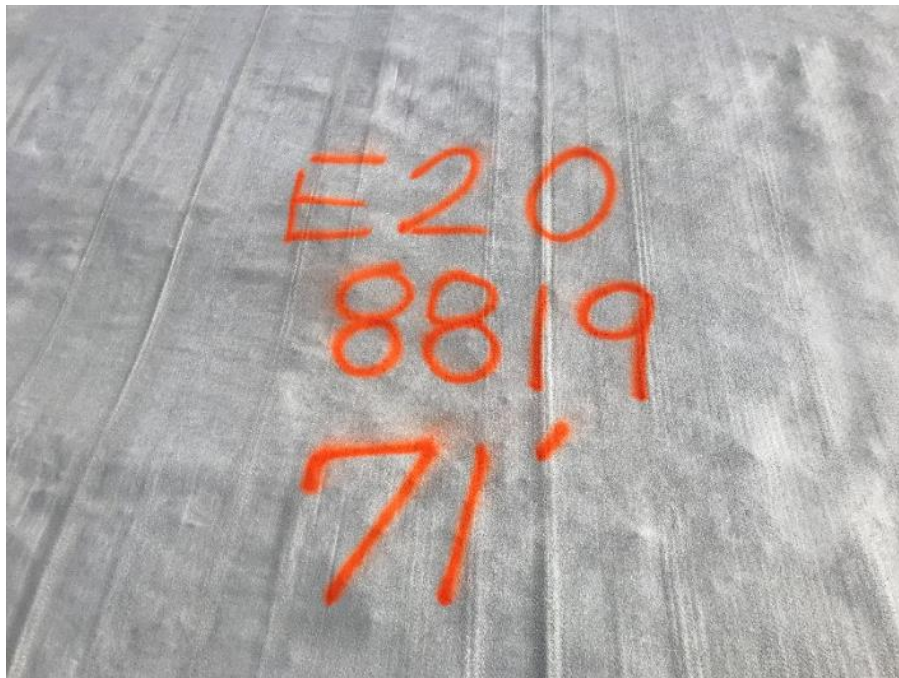
11-13-18 Installed GCL with panel number, roll number, and length marked.
