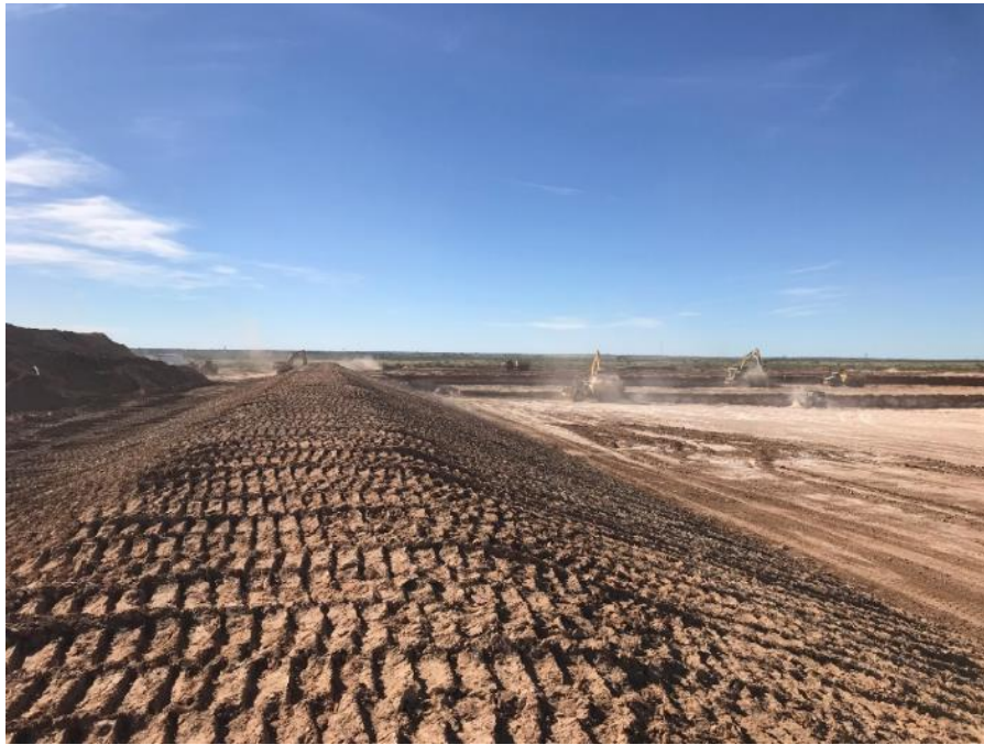
11-05-18 Southern berm construction nearing completion. West view.
