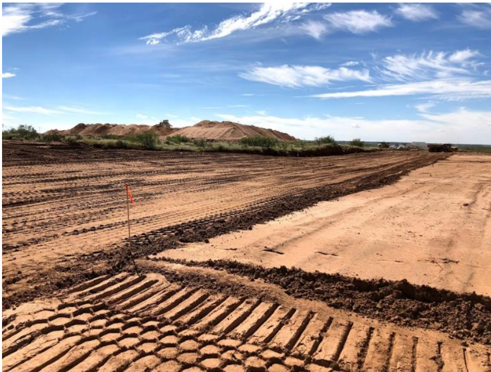
10-01-18 Area cleared, staked, and ready for berm construction. Southwest view.
