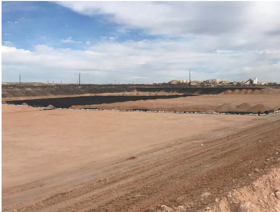
12-12-18 Protective Soil Layer installation in progress. Northeast view.
