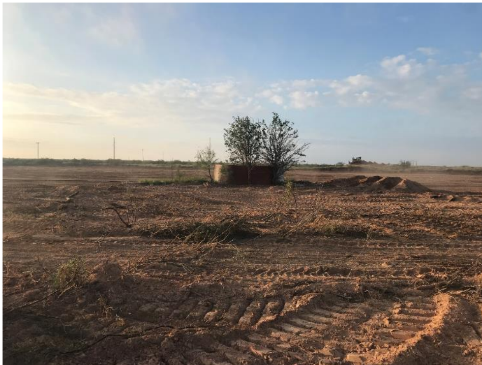
9-19-18 Unused tanks to be removed from the project area. North view.
