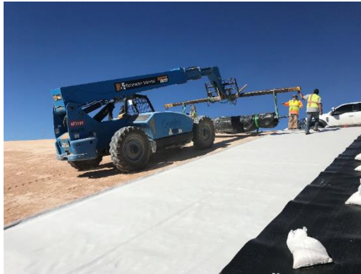
11-16-18 GCL installation in progress, north slope/berm. Northwest view.
