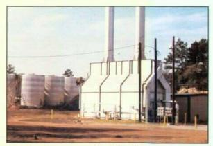
Main heating system capable of 20 million BTU's per hour.
