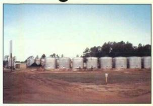
Thirty heated and insulated tanks keep material in different stages of processing.
