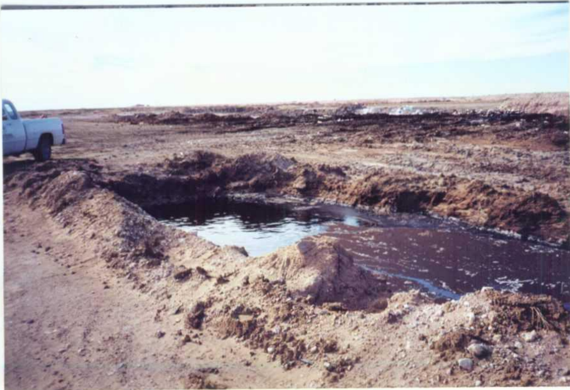
NMOCD: ID#. 831317 By: W Price #10 Date/Time: Feb 26, 1998 3pm Site/Co. CRI-Landfill OCD 711 facility Location: Landfill east of Treat Plant. Subject: Liquid unlined pit. Looking NW Bkgd shows landfill.
