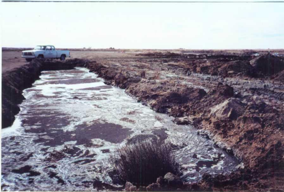
NMOCD: ID#. 831317 By: W Price #11 Date/Time: Feb 26, 1998 3pm Site/Co. CRI-Landfill OCD 711 facility Location: Landfill east of Treat Plant. Subject: Liquid unlined pit. Looking west. approx. 50 yds from landfill.
