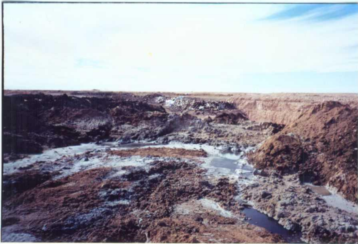
NMOCID: ID#, 831317 By: W Price #12 Date/Time: Feb 26, 1998 3pm Site/Co. CRI-Landfill OCD 711 facility Location: Landfill east of Treat Plant. Subject: SE corner of landfill looking NW. Waste with free liquid near edge.
