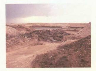
Photo 13 May 31, 2000 Pond 3d, evaporation pond contains solids. Oily liquids have flowed between 3d and 3c thorough breach in berm.
