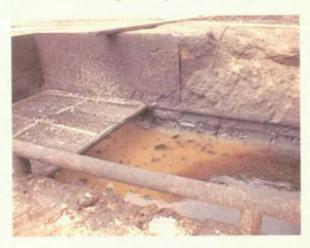
Photo 8 May 31, 2000 Pit 2a, steal jet out pit full of wash water with some oil.
