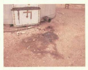
Photo 32 May 31, 2000 Tank 4, valve without sump/catchment, stained soils
