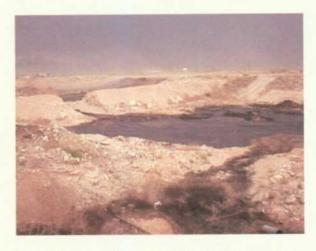
Photo 11 May 31, 2000 looking southeast Produced water evaporation pond 3c and 3d showing overflow from jet out pit.
