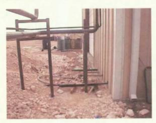
Photo 29 May 31, 2000 Boiler discharge water flowing on ground surface.
