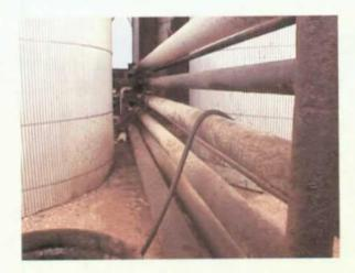
Photo 25 May 31, 2000 Treating plant pipe leaks stained soils.
