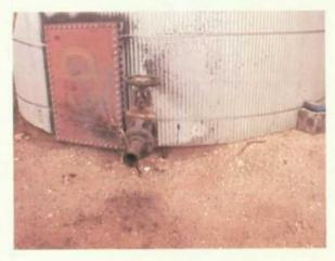
Photo 27 May 31, 2000 Tank 9, valve without sump/catchment, stained soils.
