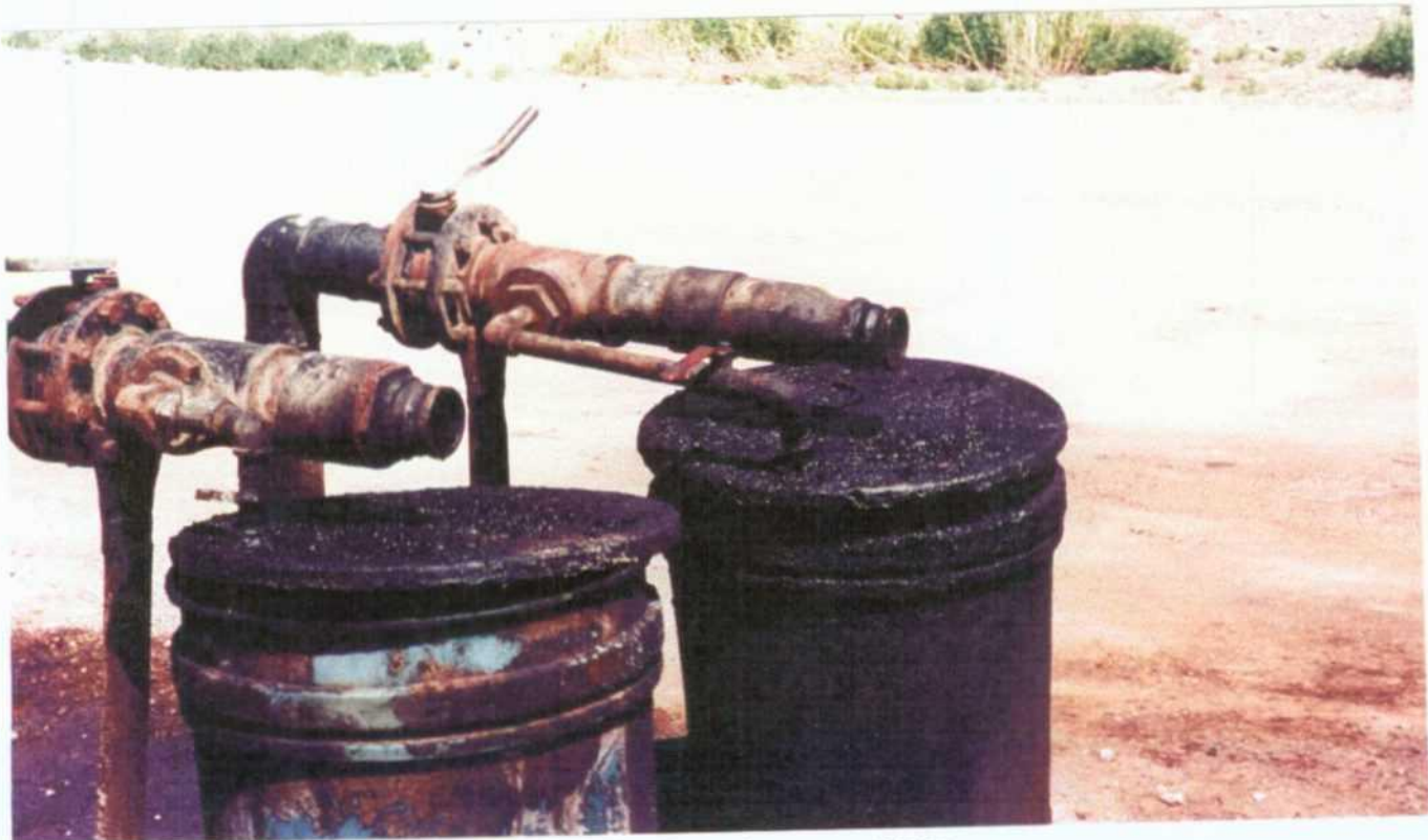
Drip Containers at SWD Note piping arrangement for emptying of container
