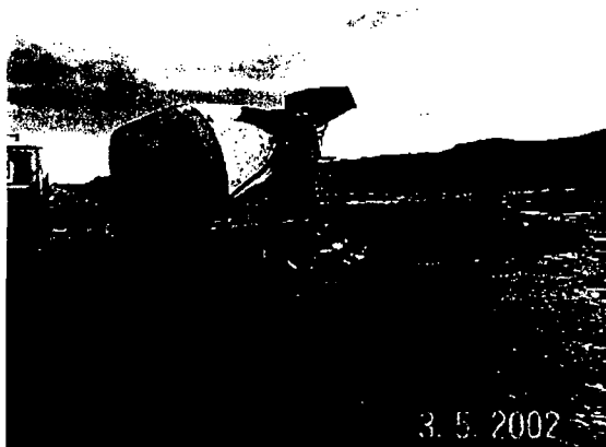
Photo 8: Mixer is solidifying sludge from the closure of the temporary pit. Material is then shipped to Tierra Environmental for landfarming.
