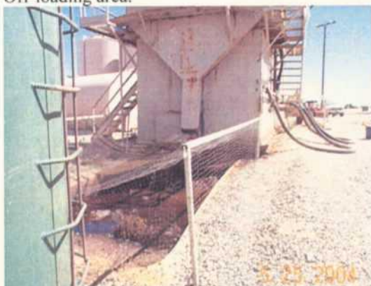
Single lined steel pit. Standing oil and water.
