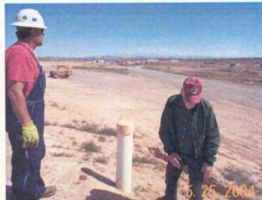
Skim pit leak detector-noted DRY.
