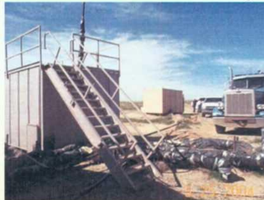
Well Pump Suction Tank and Lines.
