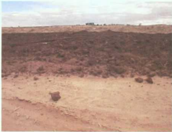
Photo 1 05-17-00 Lift thickness is greater than 10 inches.
