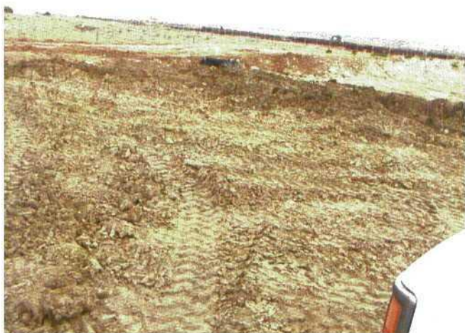
Photo 9. May 7, 2003, clearing landfarm for county road construction. Red soil is the compacted boundary berm and edge of holding pond located in the NW corner. The dark soil in the foreground is a compacted pile of contaminated soil that has been moved and is level with the containment berm.
