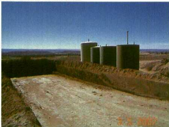
Photo 8. Concrete mixing impoundment was empty. Four unlabeled storage tanks. Tanks were not bermed or on an impermeable pad/liner. Said to be empty.
