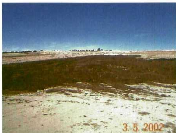
Photo 13. Material received from Basin Disposal was received to moist/sticky to be able to spread to a 10 inch thickness within the 72 hours.
