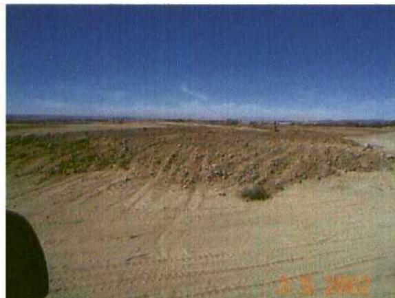
Photo 11. Soils in cell spread thicker than 10 inches
