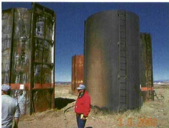
Photo 7. Tanks that have been on site for more than 6 months and are not on an impermeable liner or adequately bermed. Tanks were labeled with ID numbers but not contents.
