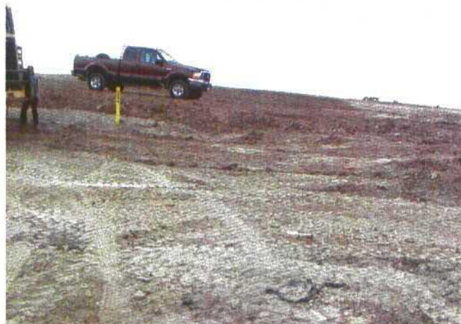
Photo 11. May 7, 2003, note plastic in the foreground and pipeline marker in the background. Contaminated soil looks to have been placed on a pipeline pathway.
