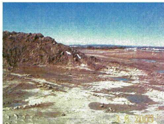
Photo 4: Pile of clean soil used to solidify sludge.
