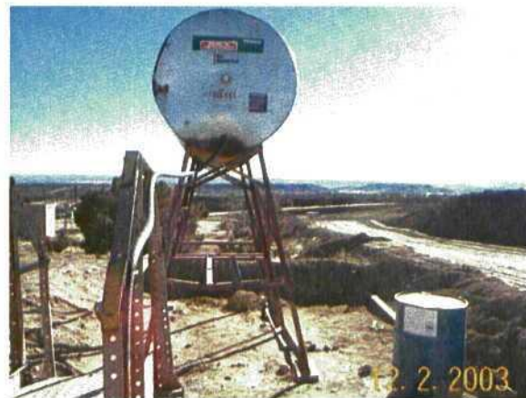
Photo 4. Fuel saddle tank is within an unlined earthen berm. The refueling hose is extended beyond the berm.
