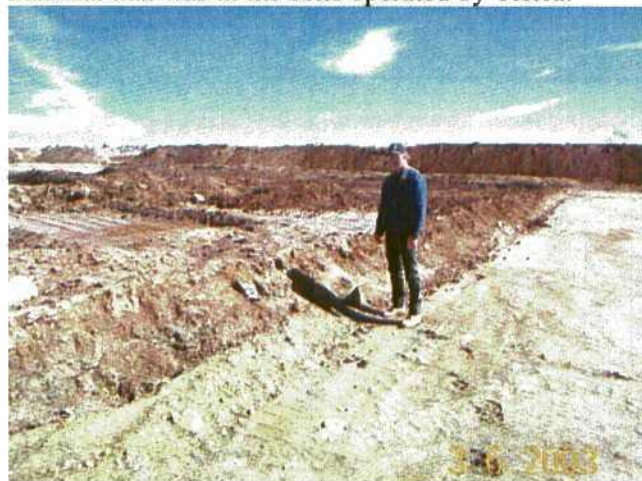
Photo 15: Landfarm cell cleared on the right. Note the thickness (2 to 3 feet deep) of the contaminated material that was in the cells operated by Tierra.
