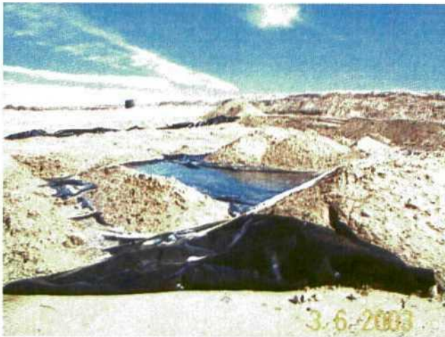
Photo 7: Construction of new tank receiving area with 30-mil liner.
