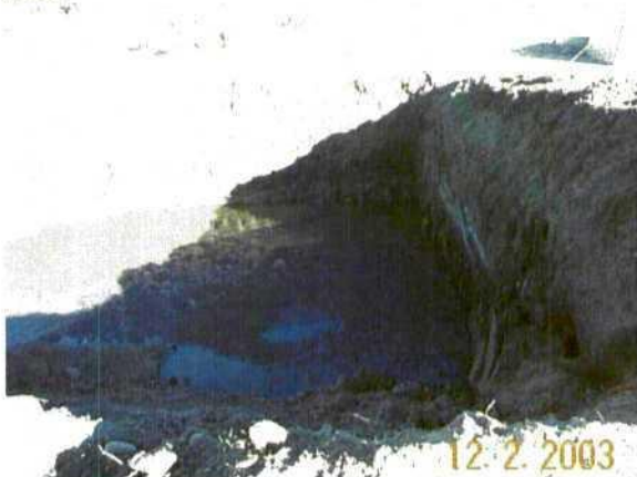
Photo 8. Concrete mixing containment has standing fluids. The wall integrity could not be determined due to the excess contaminated soil piled around the outside of the containment.
