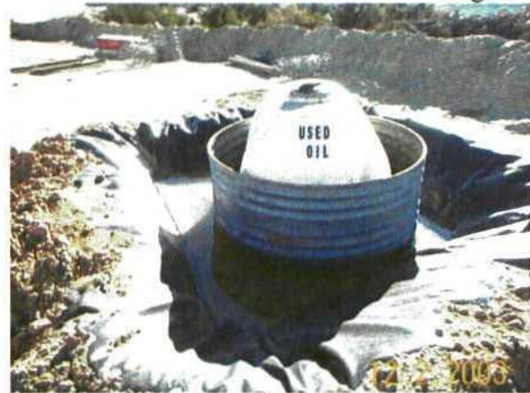
Photo 16. Used motor oil is within double containment. The water is rain/snowmelt water within the containment.
