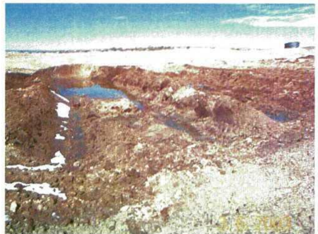
Photo 11: Landfarm cells remaining from Tierra's use; Note thickness of contaminated material.
