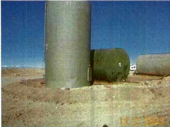
Photo 7. Tanks are bermed however the volume of the containment area does not appear to be able to contain 1 1/3 the volume of the largest tank.
