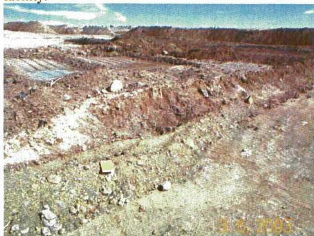
Photo 14: Landfarm cell cleared on the right. Note the thickness (2 to 3 feet deep) of the contaminated material that was in the cells operated by Tierra.
