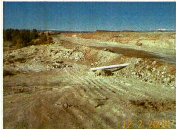
Photo 12. Storm water containment along the edge of the landfarm contains a drain pipe that releases storm water runoff directly to a natural drainage.
