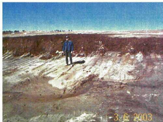
Photo 22: Landfarm cell cleared on the right. Note the thickness (2 to 3 feet deep) of the contaminated material that was in the cells operated by Tierra.
