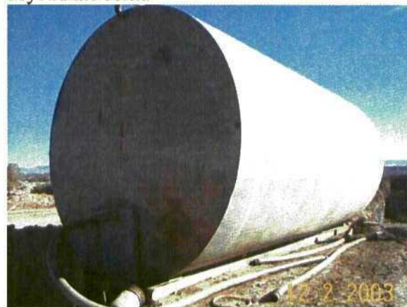
Photo 5. Tank is not labeled as to contents and is not adequately bermed to hold 11/3 the volume of the largest tank.
