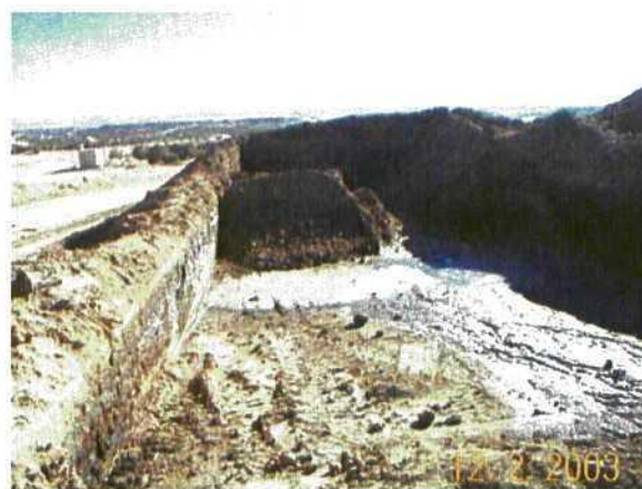
Photo 6. Concrete mixing containment is has standing liquid. The outside walls are covered and are not accessible for inspections.
