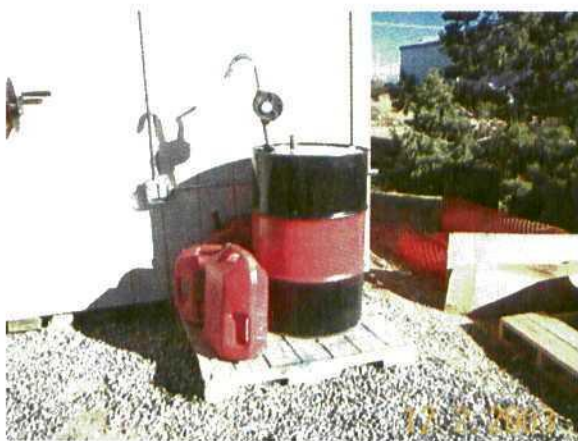
Photo 2. Fuel / oil is not within an impermeable berm or containment.
