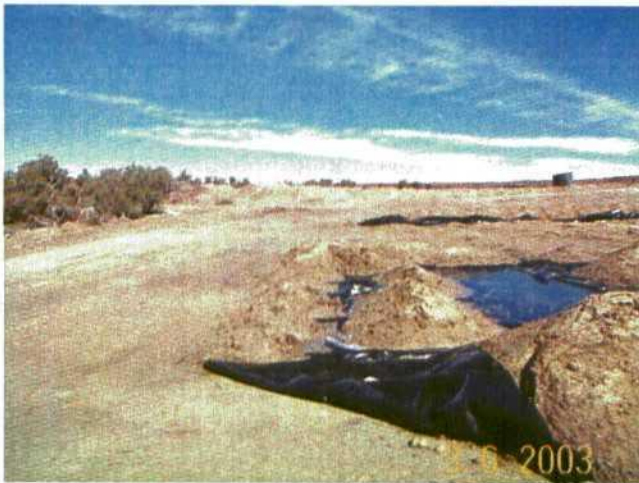
Photo 8: Construction of new tank receiving area with 30-mil liner.
