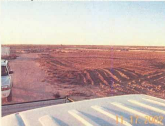
Photo 7. Landfarm cells have been tilled. Berms are worn down.
