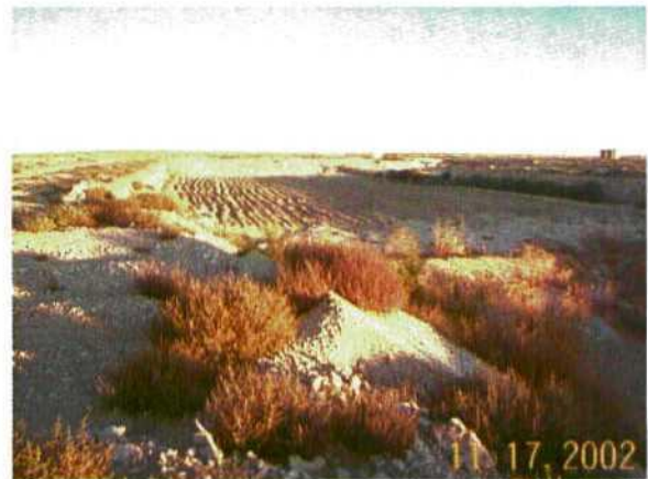
Photo 5. The landfarm cell has been tilled and the berms are in good conditions.
