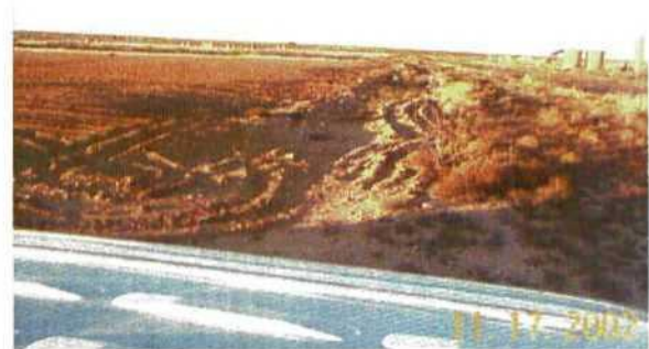
Photo 6. Berms surrounding the landfarm cell have been eroded.
