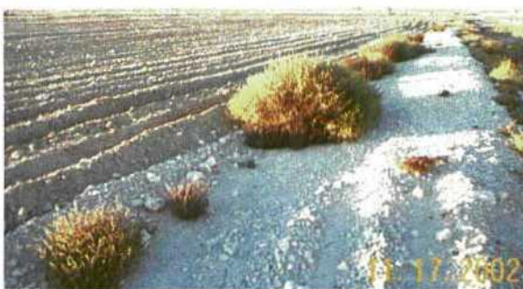
Photo 3. Berms surrounding the landfarm cell have been eroded.
