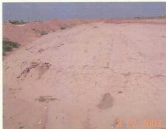
Photo 5: Cell #? next to dosed house. Lift thickness looks to be approximately 2 to 2.5 feet. This is greater than the 8 inches allowed in the permit. The gray spot in the bottom center of the photo is a boot print for scale on the sloped front of the lift. Looking west.
