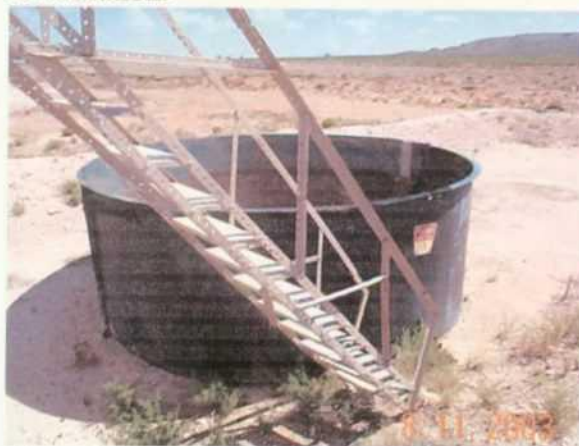
Photo 9: Netting must be repaired and reattached to the open top tank. New labels are required. Looking northeast.
