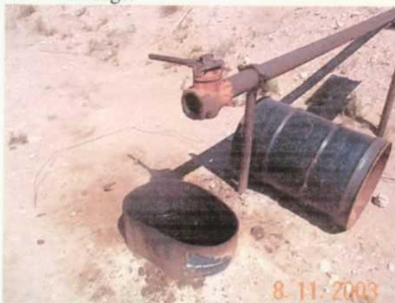
Photo 8: Drips and spills must be picked up and removed to a landfarm cell for remediation.
