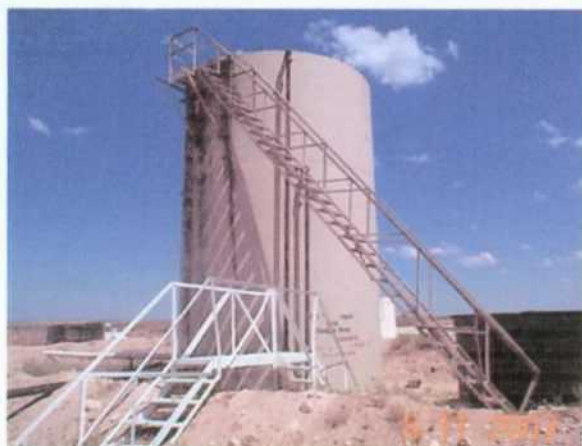
Photo 7: 750 bbl tank requires new labels regarding contents and hazards including H 2 S warnings.
