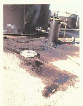
Photo 5: Oil on the ground still leaking from the tank.
