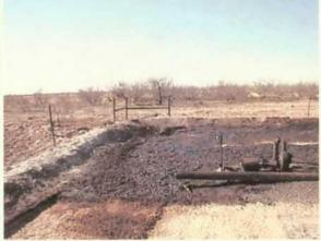
Photo 7: The southeast corner of the facility showing former berm height and fire damage well outsde the fence line to the east and south.
