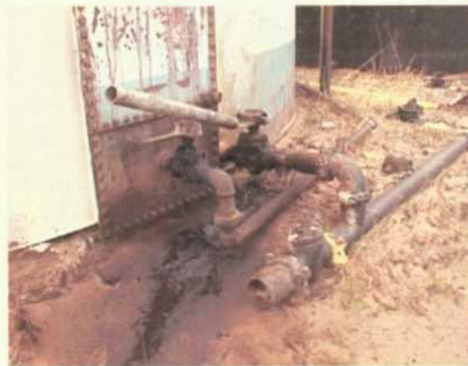
Photo 12 04-11-00 Leaking valve or pipe.
