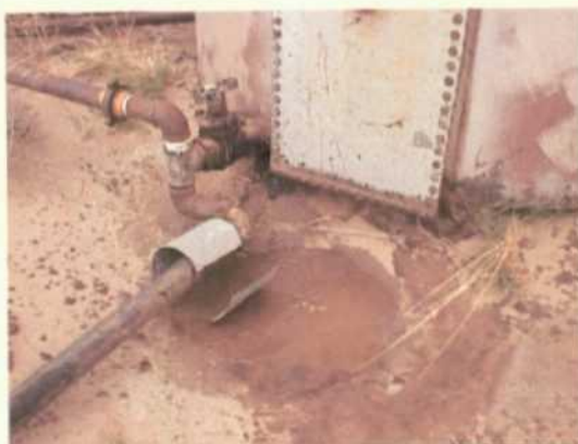
Photo 14 04-11-00 Leaking valve or pipe
