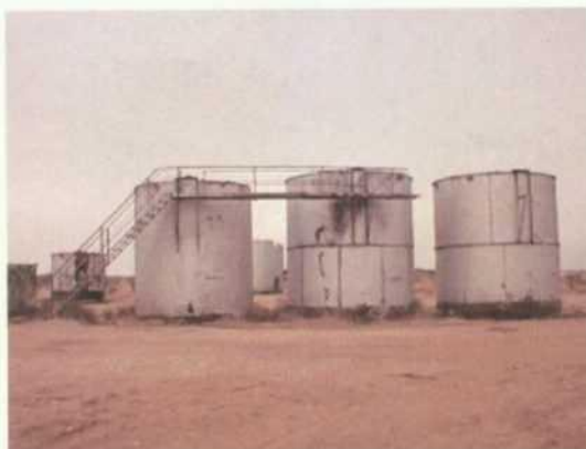
Photo 7 04-11-00 Bolted tank to be cleaned and removed
